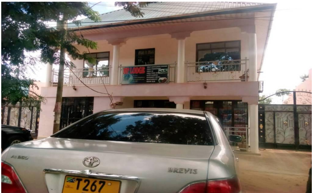
Picture No.17. MP Guest House in Tunduru Town
