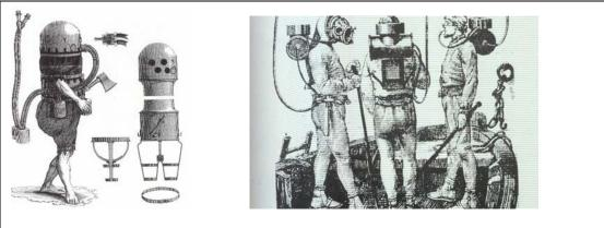
Figure 5. To the left Klingert's diving gear from 1797, and to the right, Rouquayrol and Denayrouze semi-selfcontained UBA and suit 1865. Scans from: Bachrach. A pictorial history of diving, 1988.
