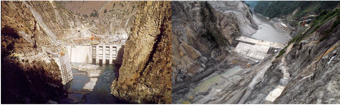
Figure 6: Degradation and Siltation in Chenab River near Dul-Hasti HE Project
