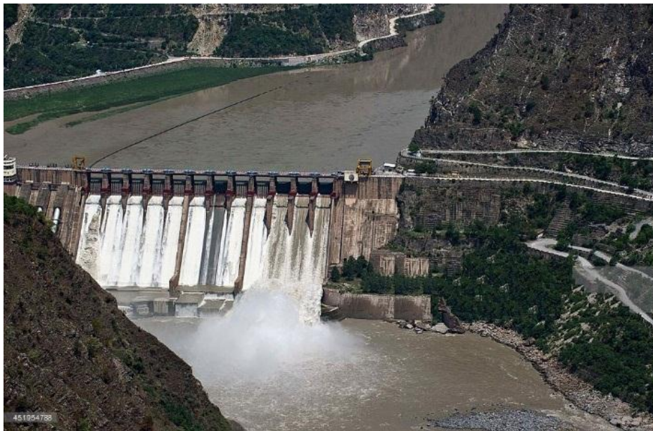
Figure 4: Ponding and dam structure of the Salal HE project
