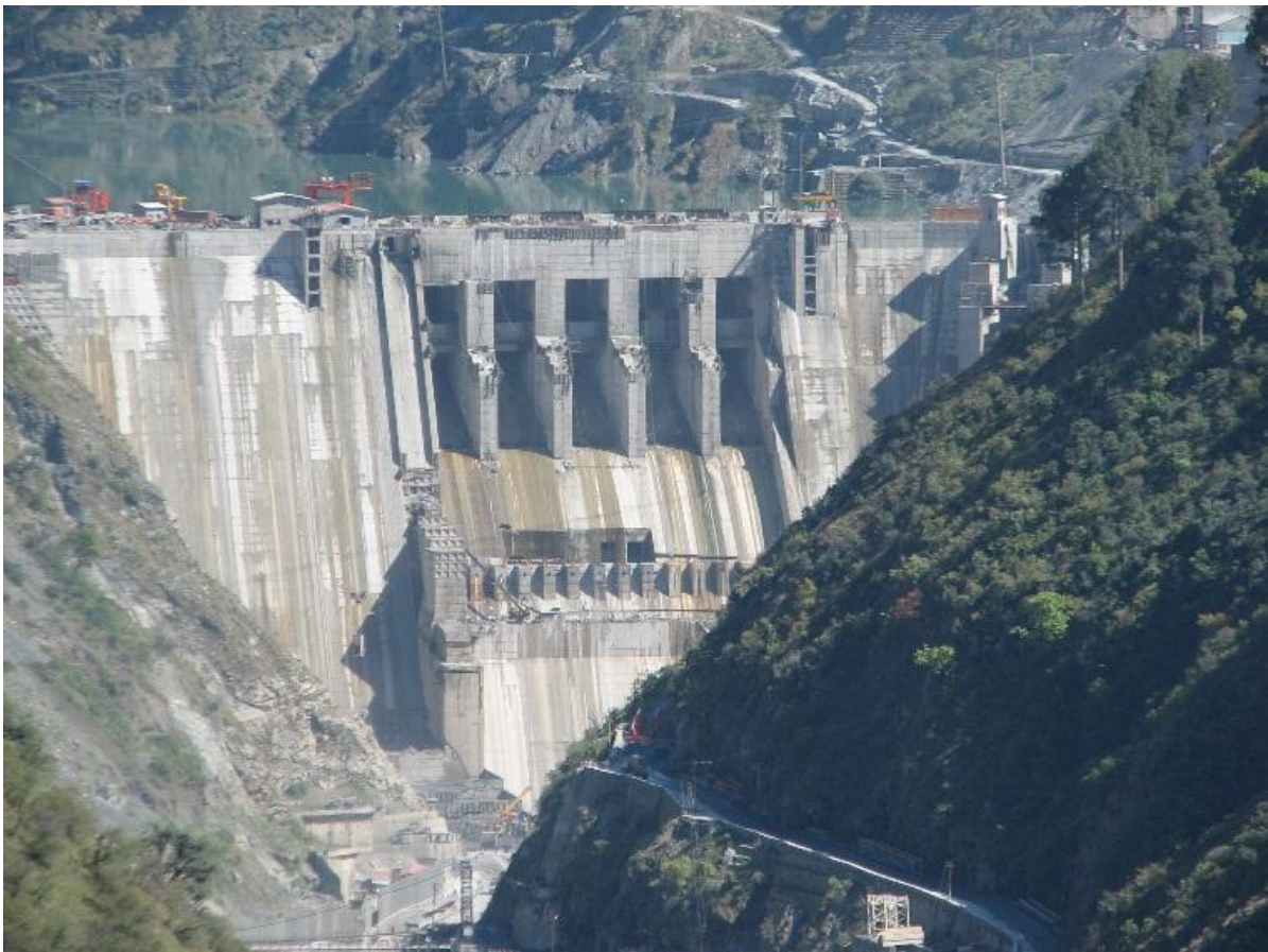
Figure 2: Ponding of the Run-of-the-River Baglihar project
