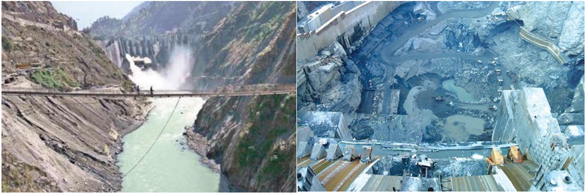
Figure 3: Chenab River bank erosion and siltation near Baglihar HE Project
