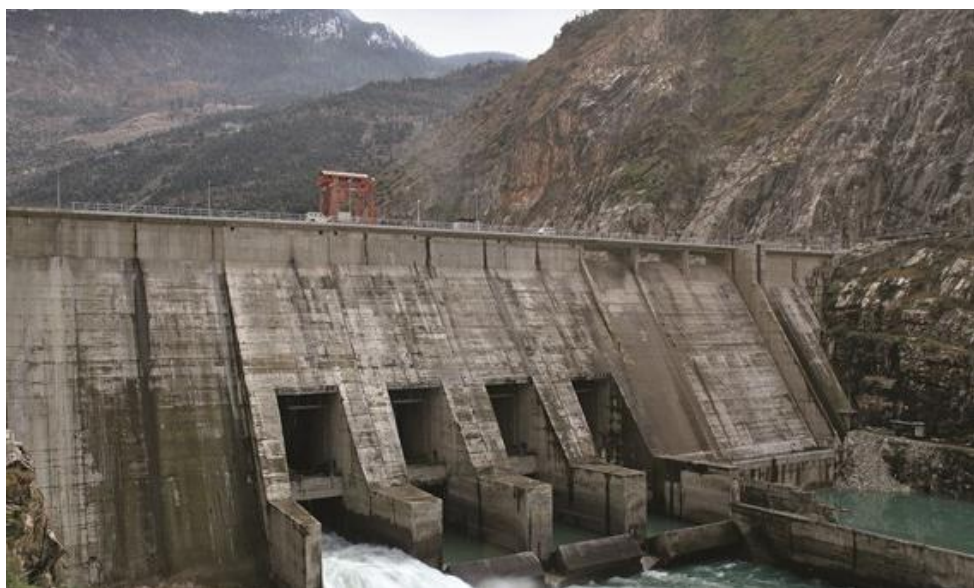
Figure 5: Ponding and dam structure of the Dul-Hasti HE project
