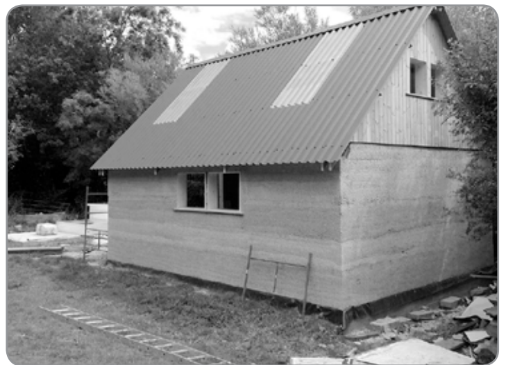
The hemp-laden fruits of a summer well spent! The walls of the workshop are made from hemp and lime – a greener approach to construction.
