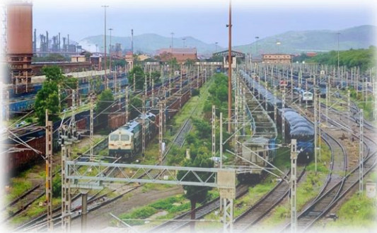
Raw Material Receipt Yard
