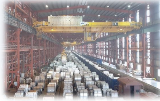
Cold Rolling Mills Dispatch
