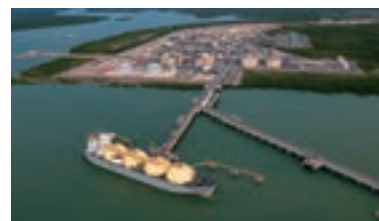
Ichthys onshore production plant
