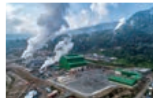
Muara Laboh Geothermal Power Project
