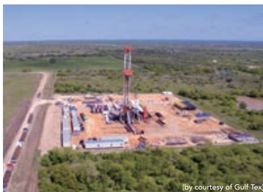
Drilling operations site
