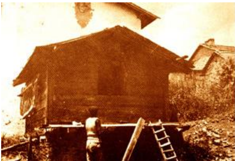
Figure 2.7.3. Horizontal wooden depot
