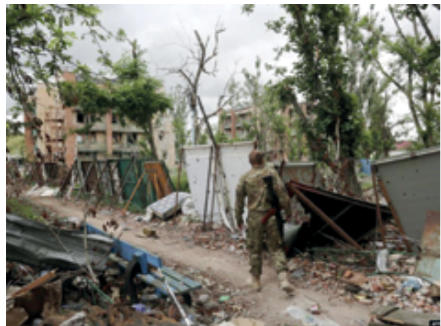
Photo 19. Protective structures of the Ukrainian military in the village, Shyrokyne, 2015. Source: Anatoliy Stepanov Facebook page
