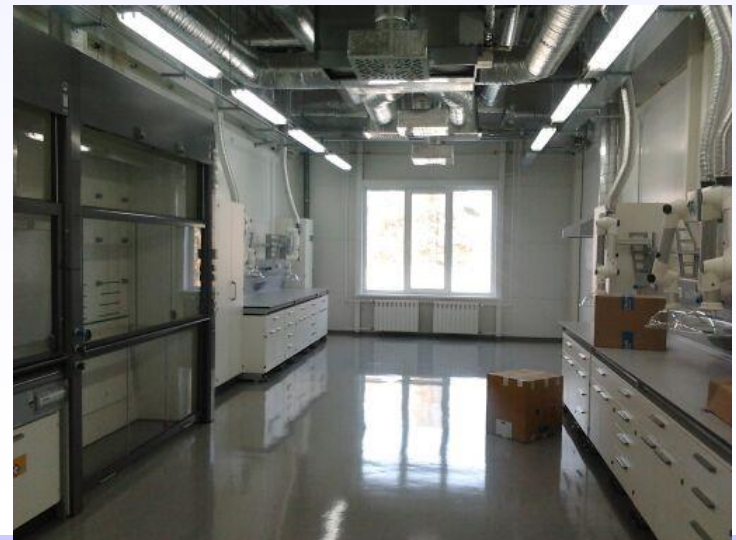
Centre of Nanotechnology, interior view
