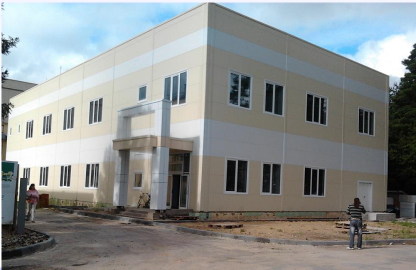
General view of the new laboratory building (Centre of Nanotechnology)
