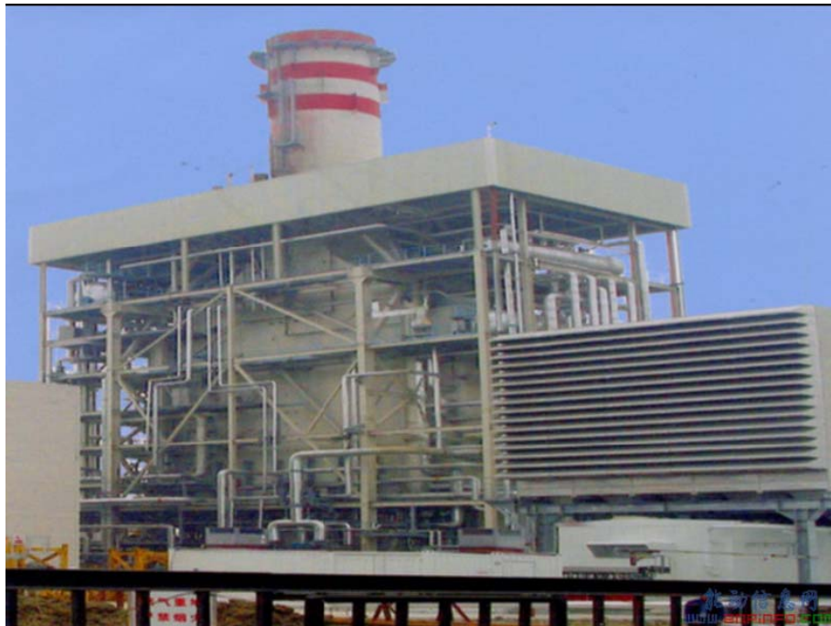
Figure 3: General Electric (GE) MS9001E Gas Turbine Combined Cycle Unit
