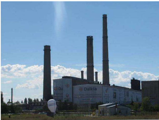
Brazi power plant
