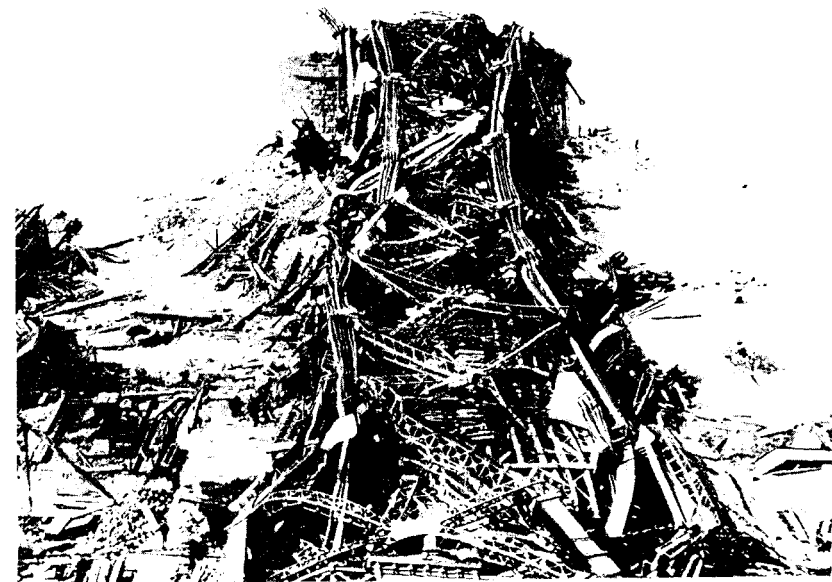
Fig. 9.2 Quebec Bridge after collapse.
