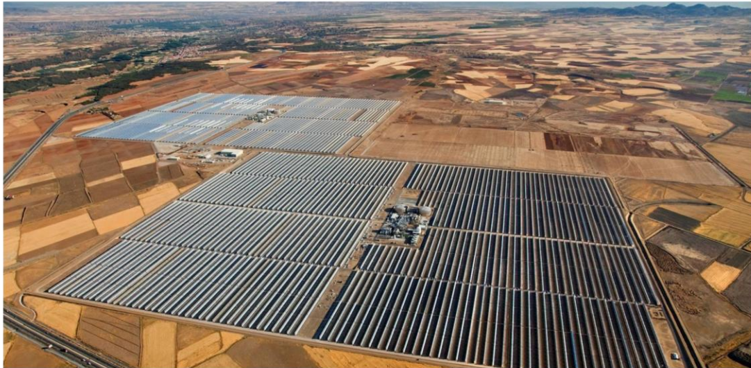
Figure 1: Parabolic power plants in southern Spain (Andasol 1 and 2, in the back ground on the right side the prepared construction ground for Andasol 3, source: Solar Millenium)
