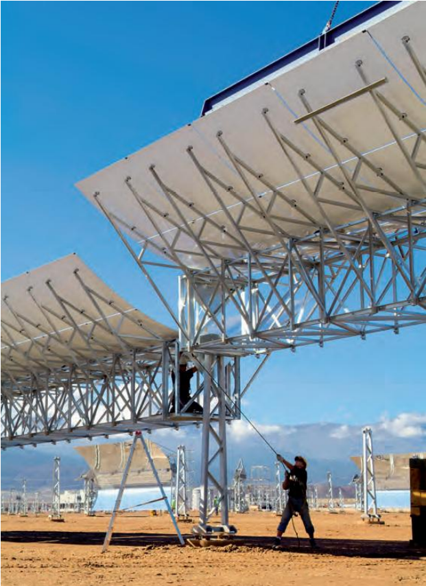
Figure 24: Mounting of the Eurotrough collector to the pylon (source: Solar Millenium)
