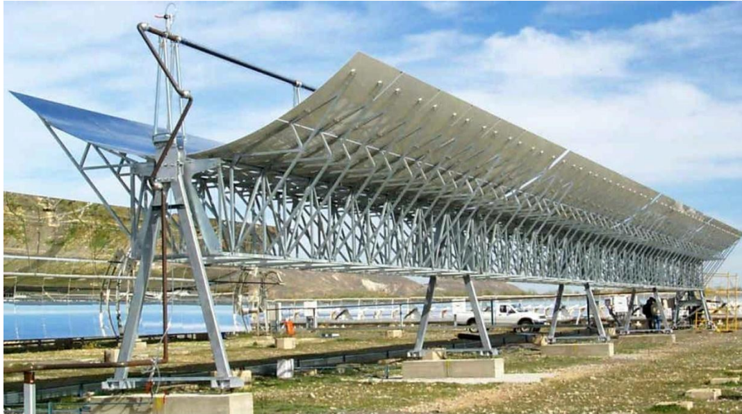
Figure 27: Eurotrough collector, test facility at the PSA (source: Lüpfer, DLR)
