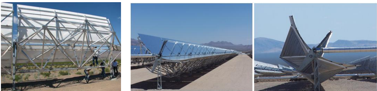
Figure 29: Solargenix collector (source: Kearney, NREL, gossamersf.com)
