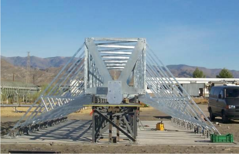
Figure 23: Assembly of the Eurotrough module with the help of an assembly jig (source: Lüpfert, DLR)
