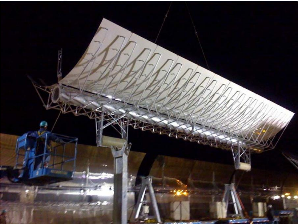
Figure 33: Installation of a Heliostroph collector element in one of the SEGS plants (source: Flagsol)
