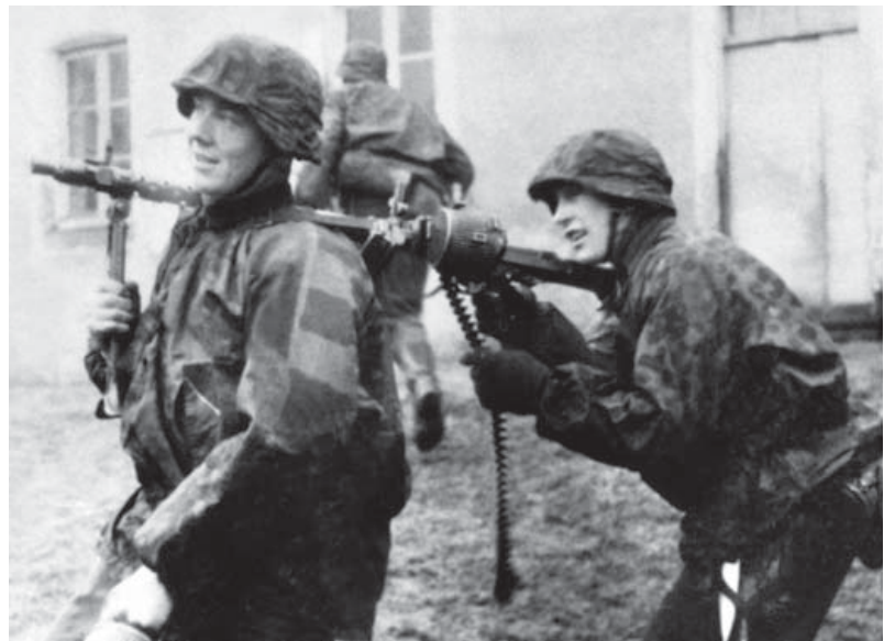
Only for the brave. This manual-taught method of mounting and firing the MG 34 placed the man at the front under appalling noise and blast from the muzzle. This MG 34 is fed from a Gurttrommel 34 belt drum. (Cody Images)
