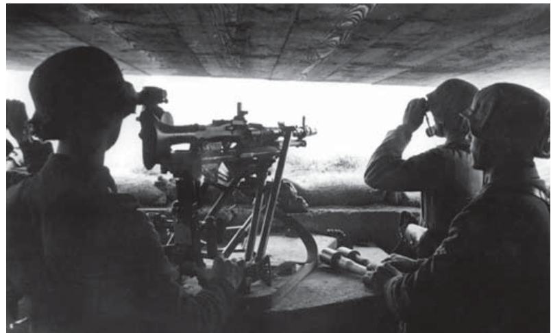
A Lafette-mounted MG 34 in an Atlantic Wall pillbox, France, 1943. The MG 34 was much better suited to fortress use than the MG 42, because its barrel-change system was more convenient for enclosed spaces. (Cody Images)
