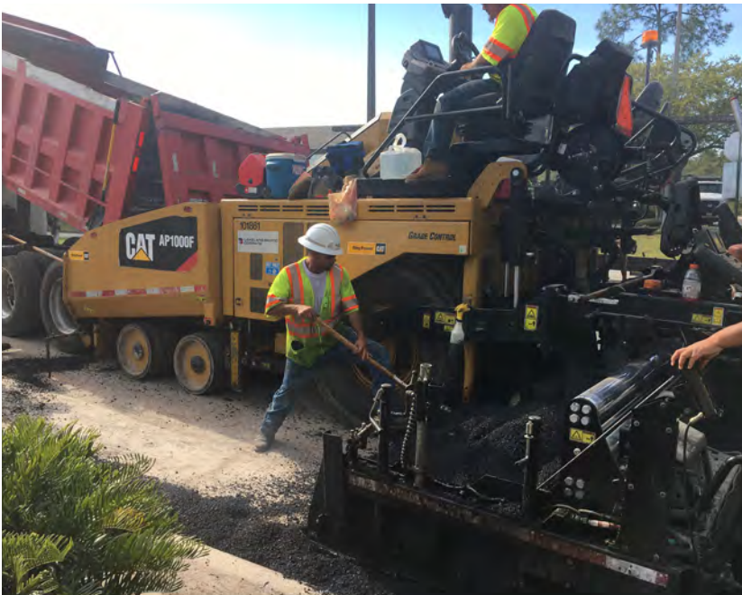
Countywide Construction Services crew workers resurface a County road.
