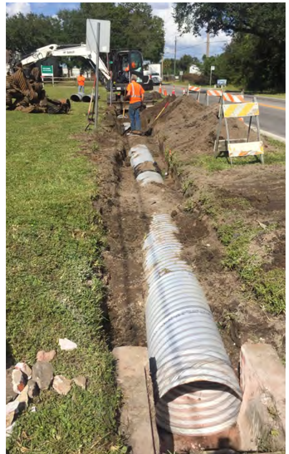
Transportation Maintenance crews repair a failing stormwater pipe
