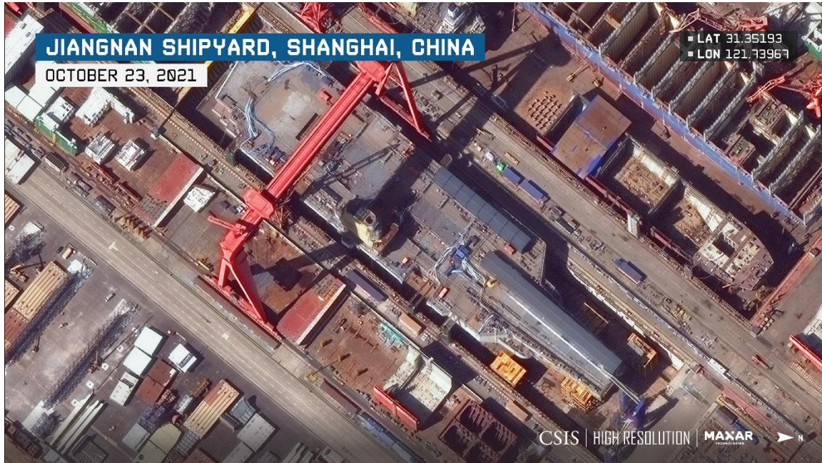
Figure 12. Type 003 Aircraft Carrier Under Construction
