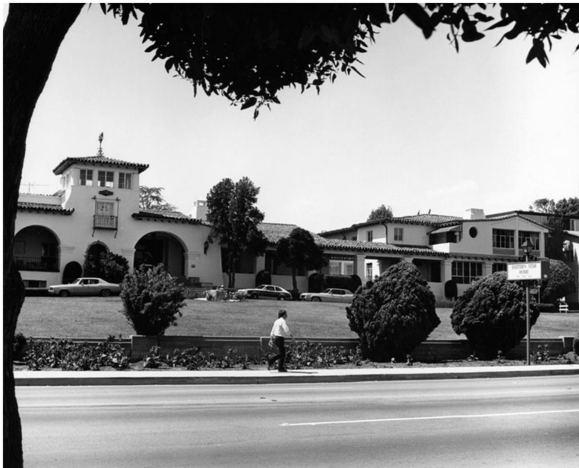
Figure 13. Eastern Star Home, 1980. Source: Los Angeles Public Library.
