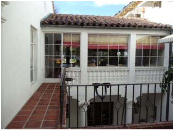
Upper story, secondary façade, Main Building.
