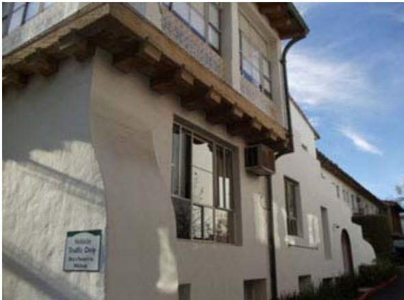
Secondary façade Main Building.
