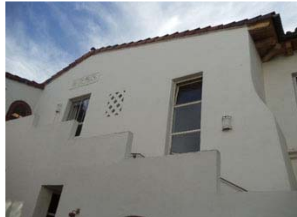
Secondary façade Main Building.
