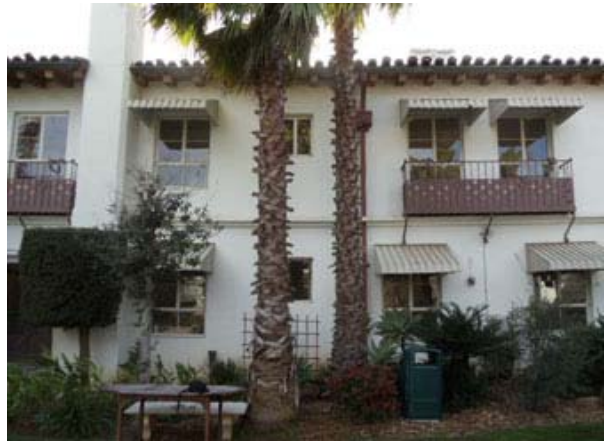
Façade of Main Building (facing interior courtyard).
