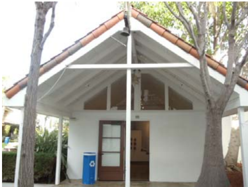
Chapel, 2011. Source: Parallax Architecture and Planning.
