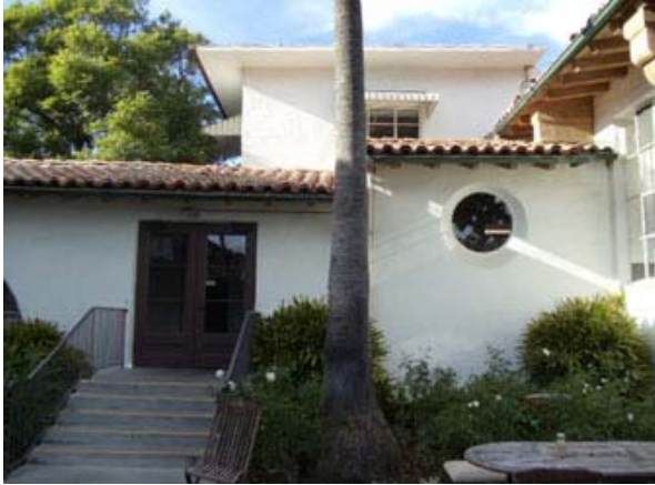
Northwest corner of courtyard; rooflines of original building and North Wing
