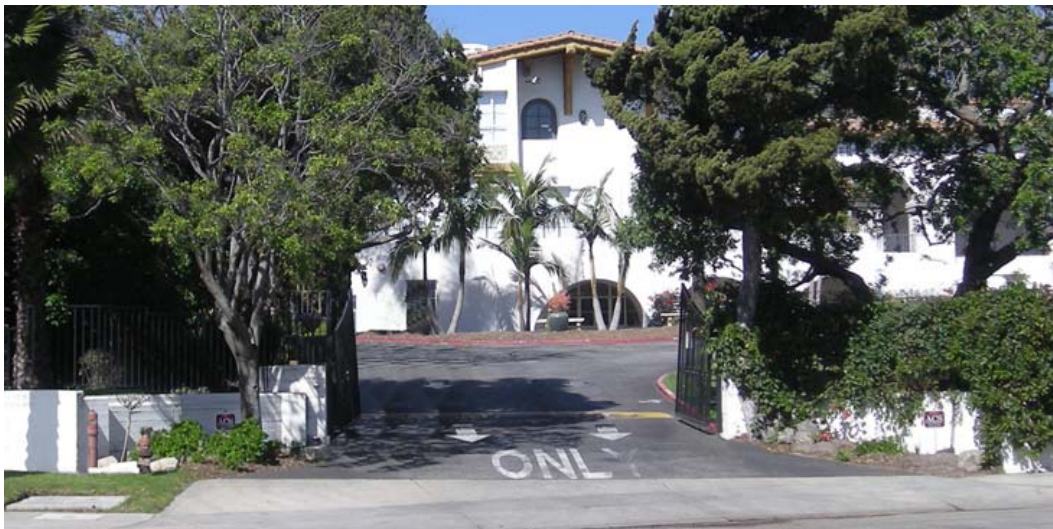
West entry after driveway widening. Source: Parallax Architecture and Planning.
