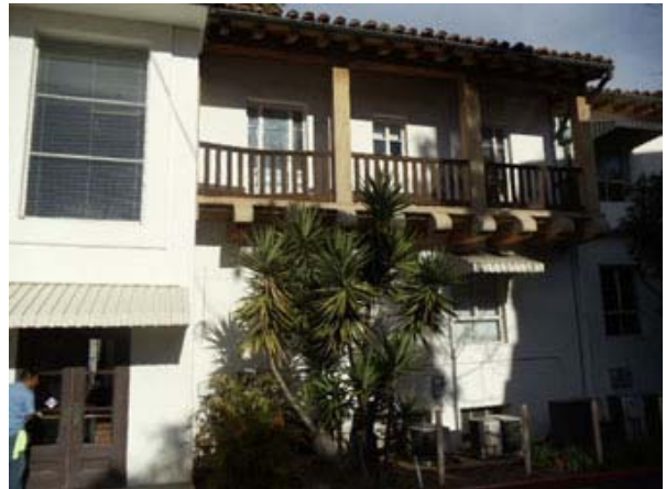
Secondary façade, Main Building.
