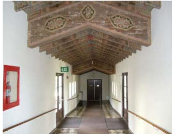
Hallway facing away from Dining Hall.
