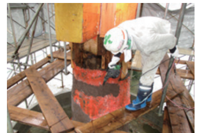
Restoration work for torii gate of Itsukushima-jinja shrine using with the restoration materials, which have evaluated in this project
