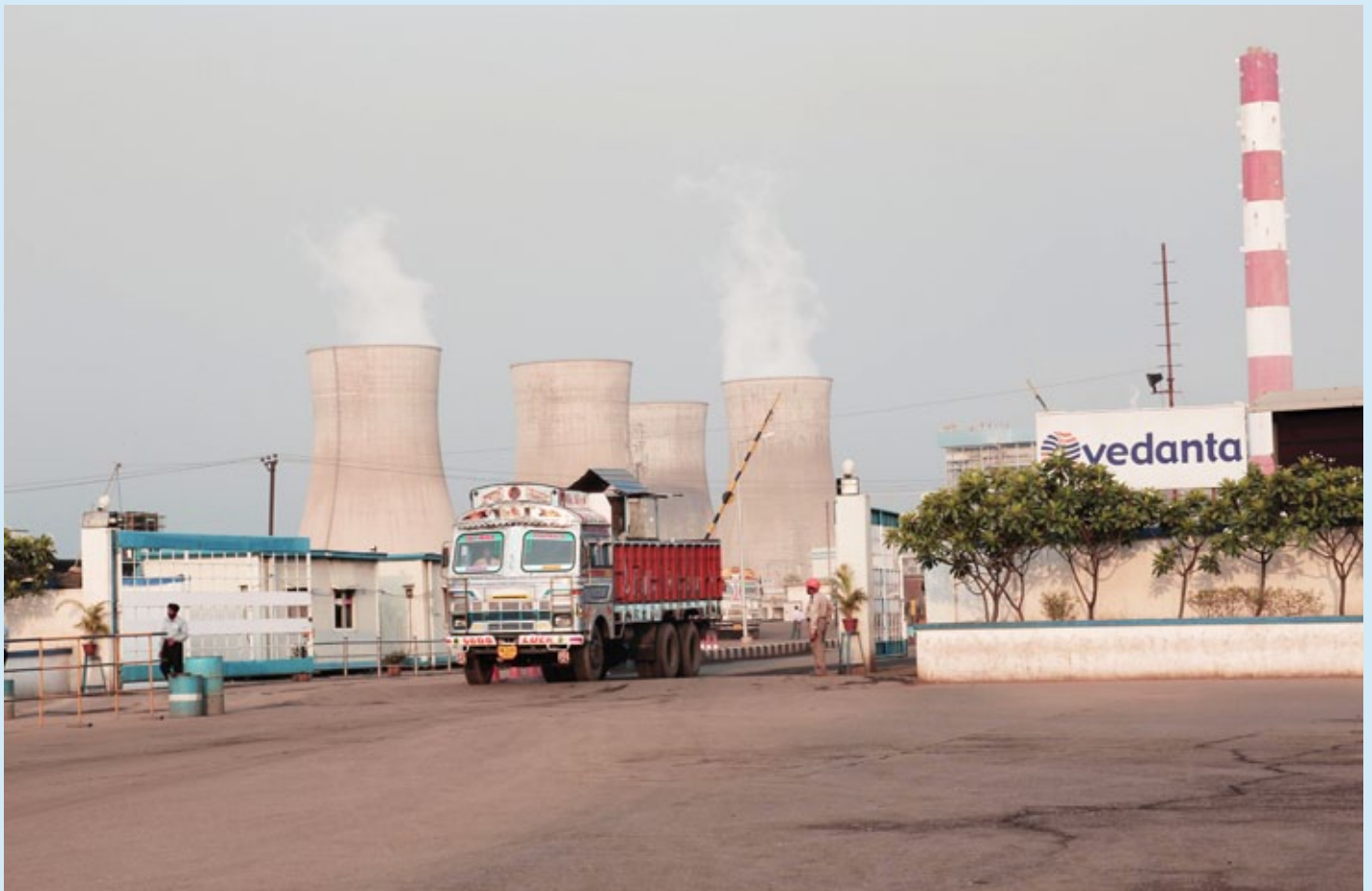
▲ Captive Power Plant (CPP) of Vedanta Aluminium Limited at Jharsuguda (Orissa) © Jenni Roth 2012
