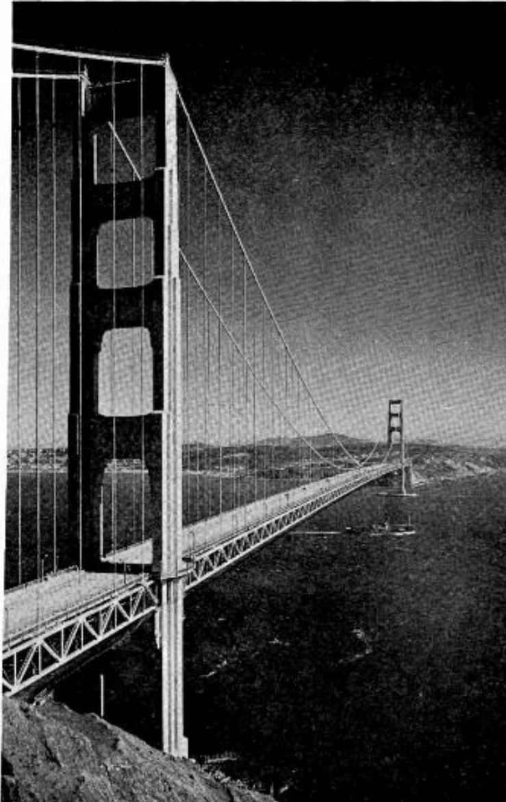
The famed Golden Gate Bridge, longest single suspension span in the world, designed by Joseph B. Strauss. Including approaches, the Golden Gate Bridge is 7 miles long. Completed in May, 1937 at a cost of $33,500,000. More than 20,000,000 cars crossed the Bridge in 1961. Photo by Moulin Studios.
