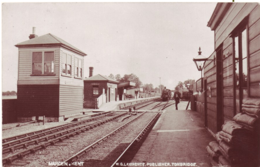
Looking down line. There was an ungated level crossing between the platforms.
