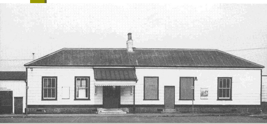
The street side of the main building, taken from the carpark
