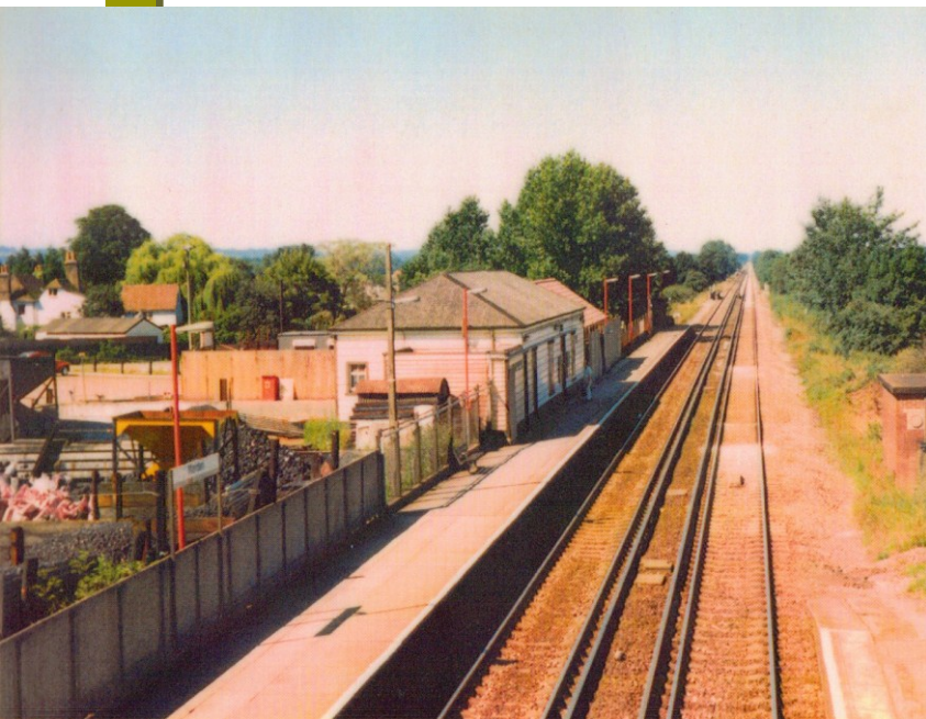
The freight sidings have, since 1960, been replaced with a goods yard that was accessed by road, then later absorbed into the growing commuter car park.
