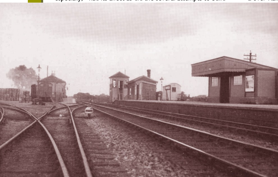
Looking up the line toward London, with freight sidings to the left (now the commuter car park)
