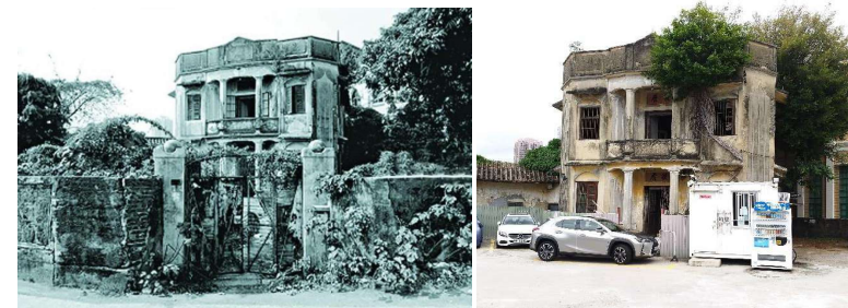
Figure 13. Siu Lo with the original entrance gate and fence wall (left) and Siu Lo in 2021 (right), (left photo: My tour, Old Hong Kong, Yuen Long, http://blog.terewong.com/archives/6304 ).
