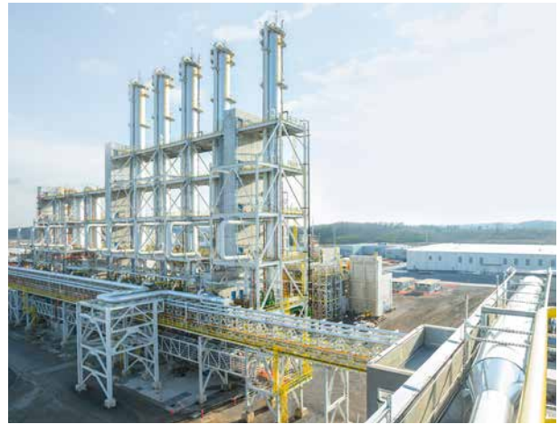
The secret of the ultrapure polysilicon lies in process control during distillation.
