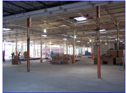
Interior view of vehicle storage area.
