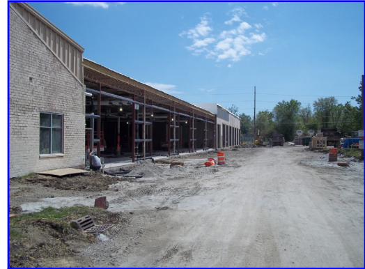
Exterior view of west side of the building.
