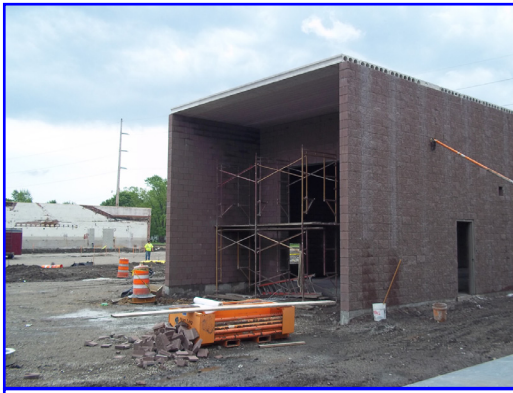
New bus wash building.
