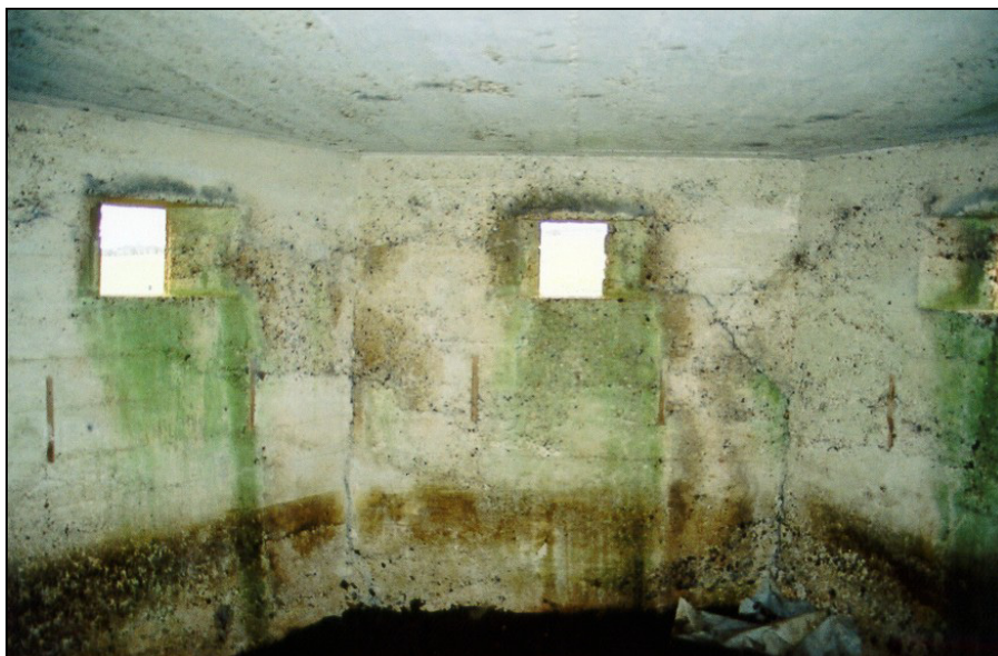
Fig. 10 - Type 22 pillbox, UORN 8224, showing one of the several cracks in its walls.
