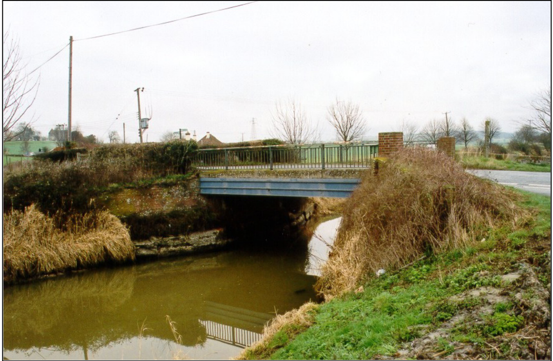
Fig. 4 - The bridge over the Canal south of Bilsington village. This bridge was prepared for demolition, whereas the one to the west at Ruckinge was actually blown up. South of both bridges were large areas of minefield and roadblocks surrounded by barbed wire.
