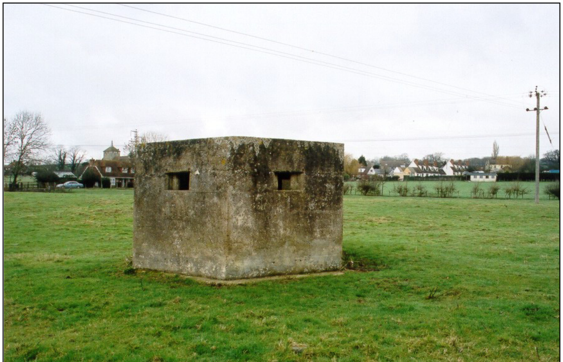
Fig. 13 - UORN 1759: the best preserved of the pillboxes in the defence area, it stands a few yards from the Canal bank at Ruckinge bridge.
