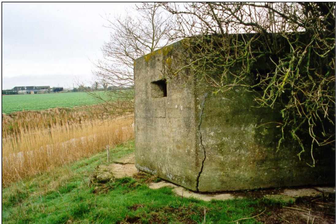
Fig. 10 - Type 22 pillbox, UORN 8224, showing one of the several cracks in its walls.
