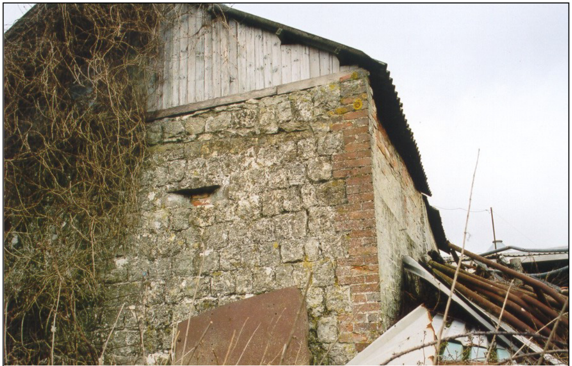
Fig. 14 - UORN 16905: blocked-up loophole in the wall of a barn. This is on a site marked 'pillbox' on the October 1940 defence map [see Fig. 6]. It guarded a roadblock.
