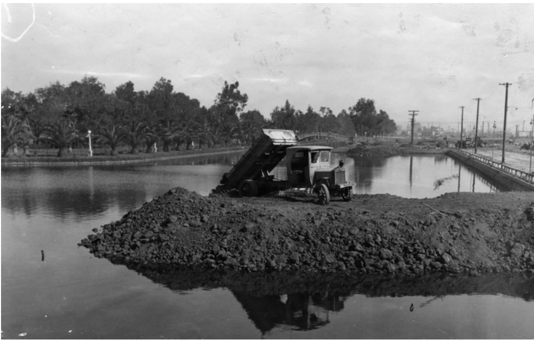
Figure 3: Filling of canals, 1927
