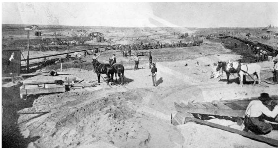
Figure 2: Dredging out marshlands, 1905
