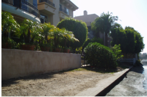
Figure 8 (right): Historic walkway along east bank
