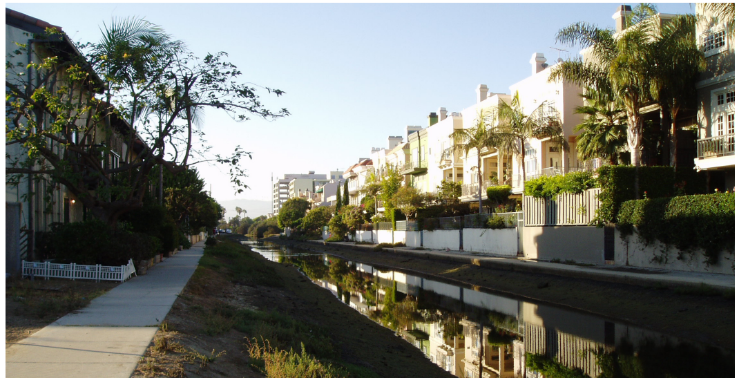
Figure 12: Concrete walkway along west bank
