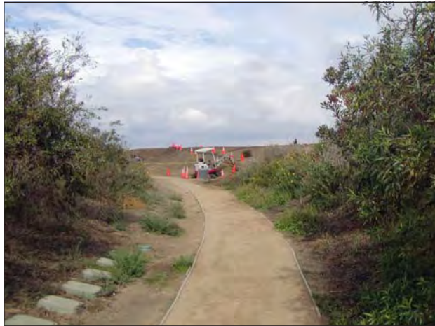
Looking west at the existing trail leading to Observation Deck
