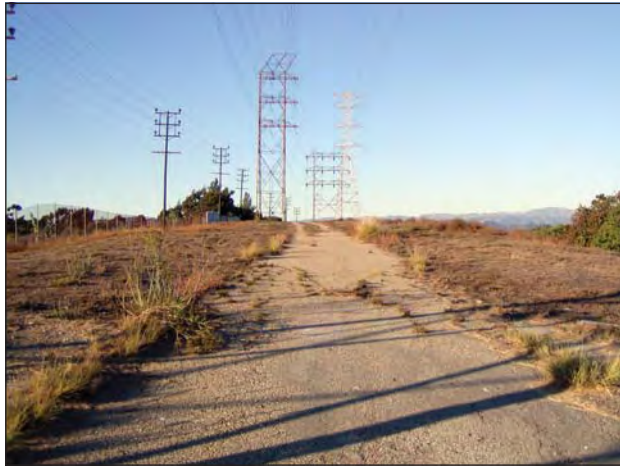
Looking north at the access road under SCE power lines
