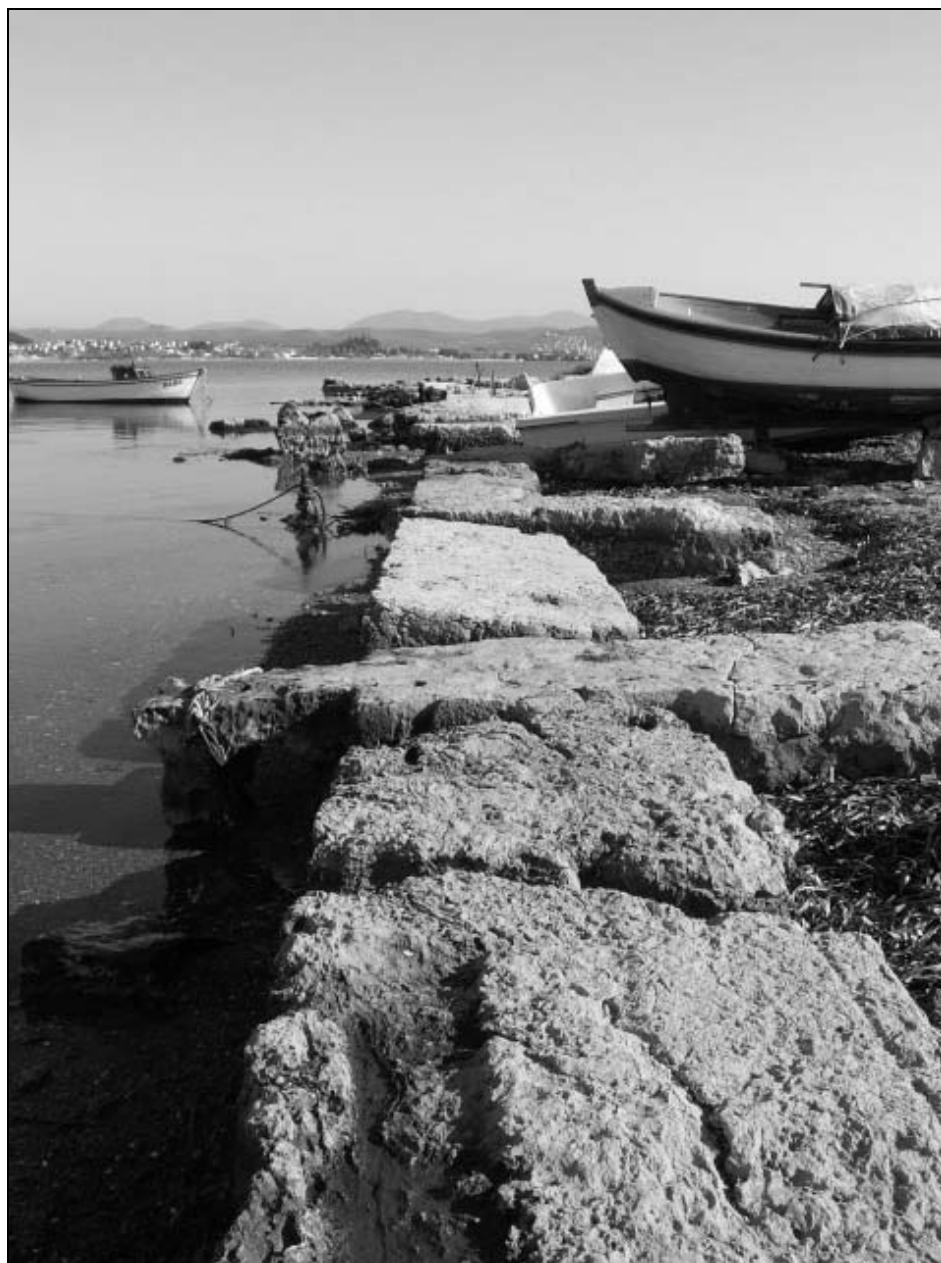
Harbor Installations, Facing East
