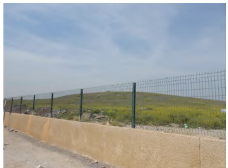
General view from the south-east with the fence.
