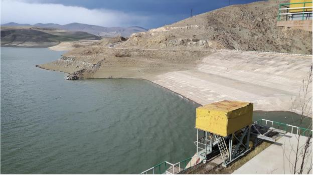
The Tolors reservoir has total capacity of 96 million m<sup>3</sup> and actual capacity 80 million m<sup>3</sup>. The water from Tolors Reservoir reaches Shamb HPP by 6.9 km long and 75 m<sup>3</sup>/sec throughput capacity tunnel.
