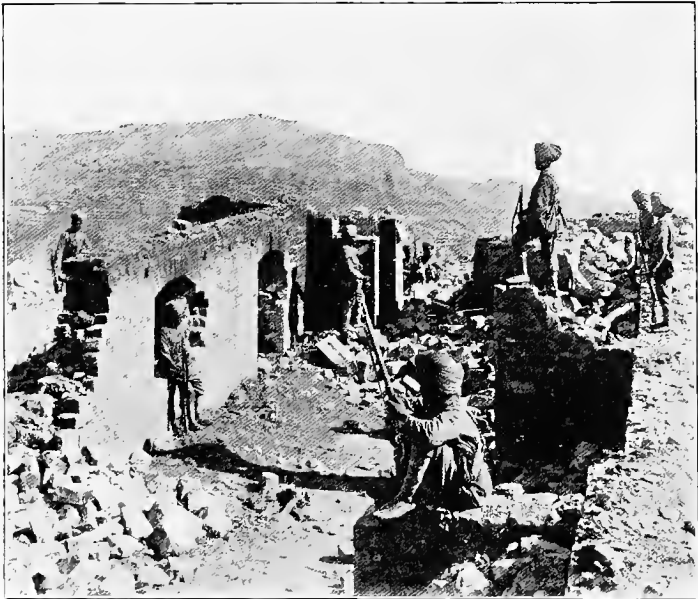
FORT SARAGARHI IN RUINS, SHOWING THE MAIN ENTRANCE AND FORT LOCKHART IN THE DISTANCE.
