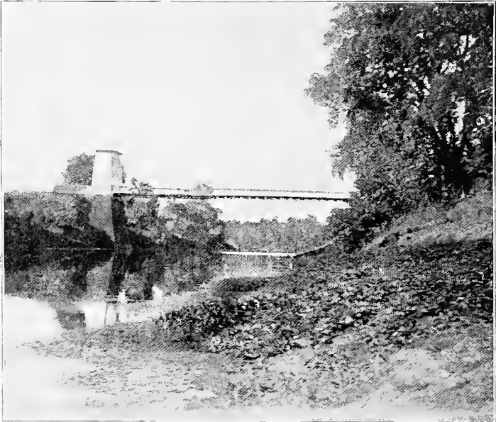
THE FIRST SUSPENSION BRIDGE IN INDIA, BUILT OVER THE BEAS RIVER BY COLONEL DUNCAN PRESGRAVE.
