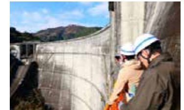
Tour of a dam and power plant in the Mimikawa River basin
