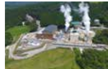
Otake Power Station
