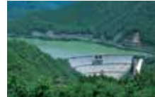
Hitotsuse Power Station
