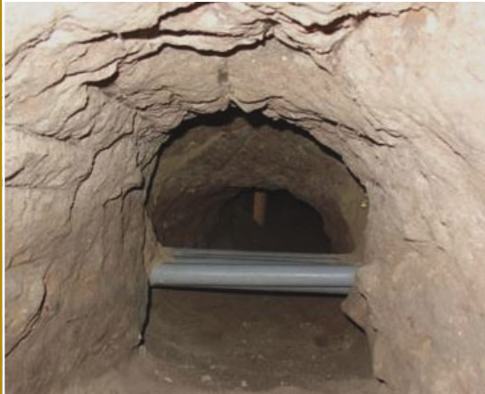
Top right: A sinkhole found in a Nogales, Arizona, street prompted officials to ask the Border Patrol to investigate, which led to the discovery of this tunnel. Municipal workers were a major source of tunnel discoveries due to smugglers' use of the city's sewer system. Two lower photos: The discovery of this tunnel, the second major San Diego-area cross-border drug tunnel to be found, led to 8 arrests and seizure of more than 20 tons of marijuana in November 2010. Two photos at left and top left: Exit and interior views depict a crudely built tunnel discovered on March 30, 2009, at Otay Mesa, California, after surveillance cameras observed a large group of suspected illegal aliens attempting to enter the country.
