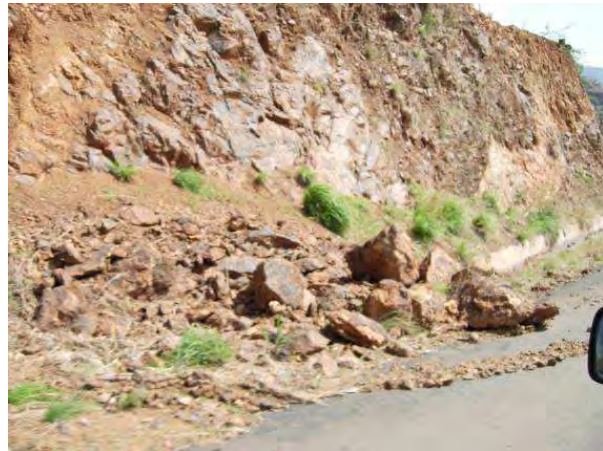
Figure III - 33 Rockfall onto the road Source, Evaluation Group photographic doc., 05.2012
