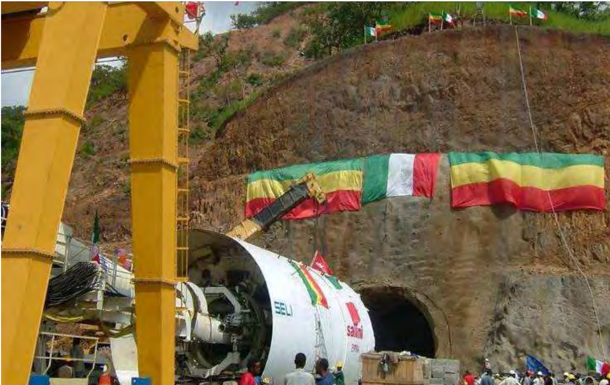
Figure II - 13: TBM 2. Outlet side works start up
