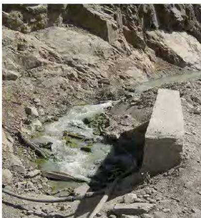
Figure III - 22: Waters discharged from the TBM excavation activity and dumped directly into the river without any processing Source: ELC, November 2006
