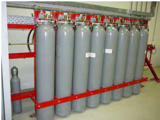
Figure II - 29: CO 2 Fire system
