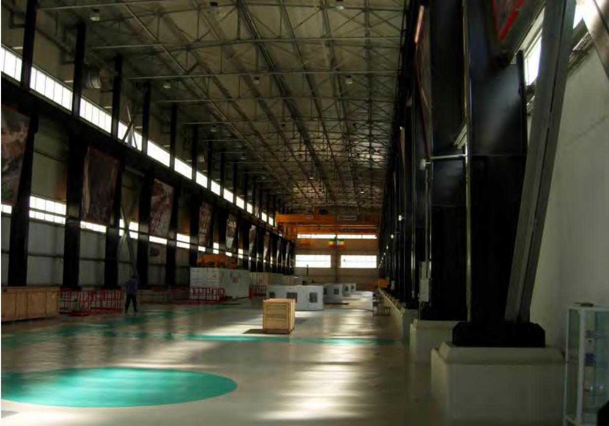
Figure II- 26: Interior of the elevated part Source: photographic documentation of the evaluation team
