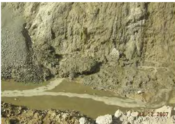
Figure III - 26: Contaminated water from the "batching plants" discharged into the river without any processing Source: ELC, December 2007
