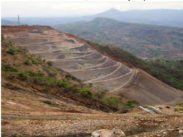
Figure III - 44: Stabilisation reprofiling of the "Disposal Area", Outlet side
