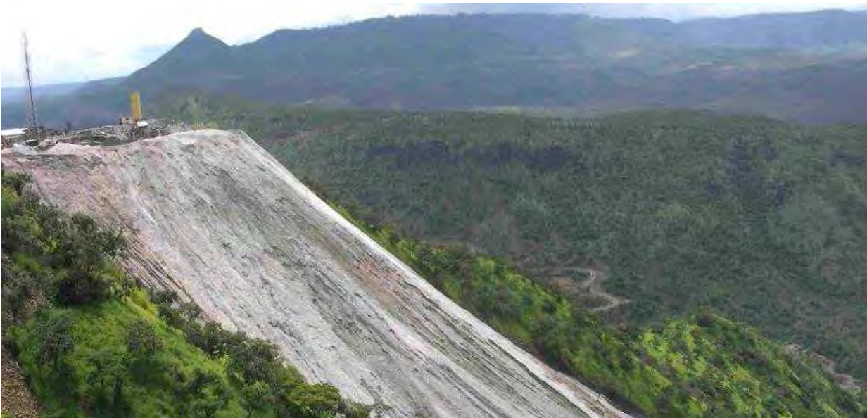
Figure III - 38: The summit of the tunnel excavation debris containment area - outlet side
