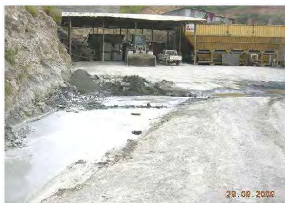
Figure III - 27: Contaminated water from the "batching plants" ends up in the river without any processing Source: ELC, October 2009
