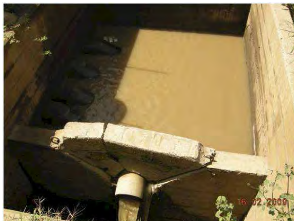
Figure III - 21: Processing unit (sedimentation only) of the waters discharged from the TBM boring activity Source: ELC, February 2009
