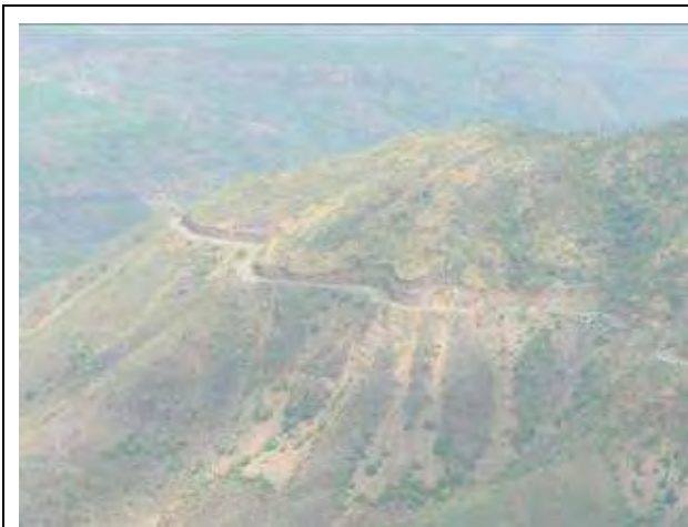
Figure II - 8: Road that from the Outlet leads to Fofa Source: photographic documentation of the evaluation team
