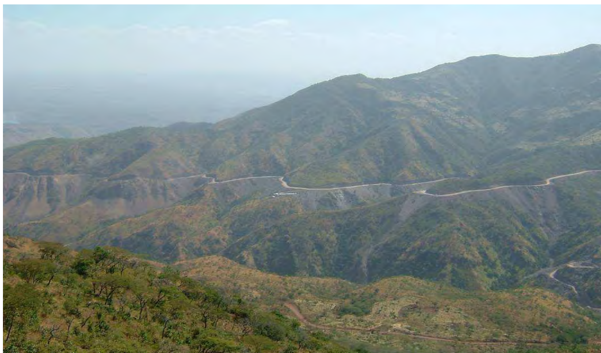
Figure III - 46: Link road between Fofa, the Outlet camp and the bridge on the Omo River Source: "A summary of the company participation in the social sphere", General Contractor
