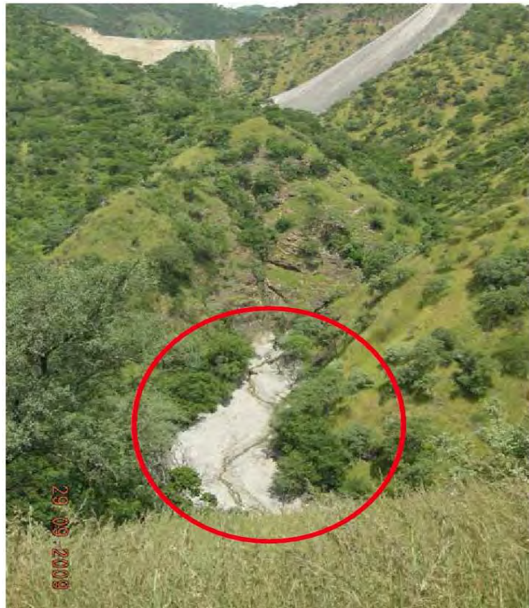
Figure III - 41: Tunnel excavation material washed away along the stream bed Source: ELC, October 2009
