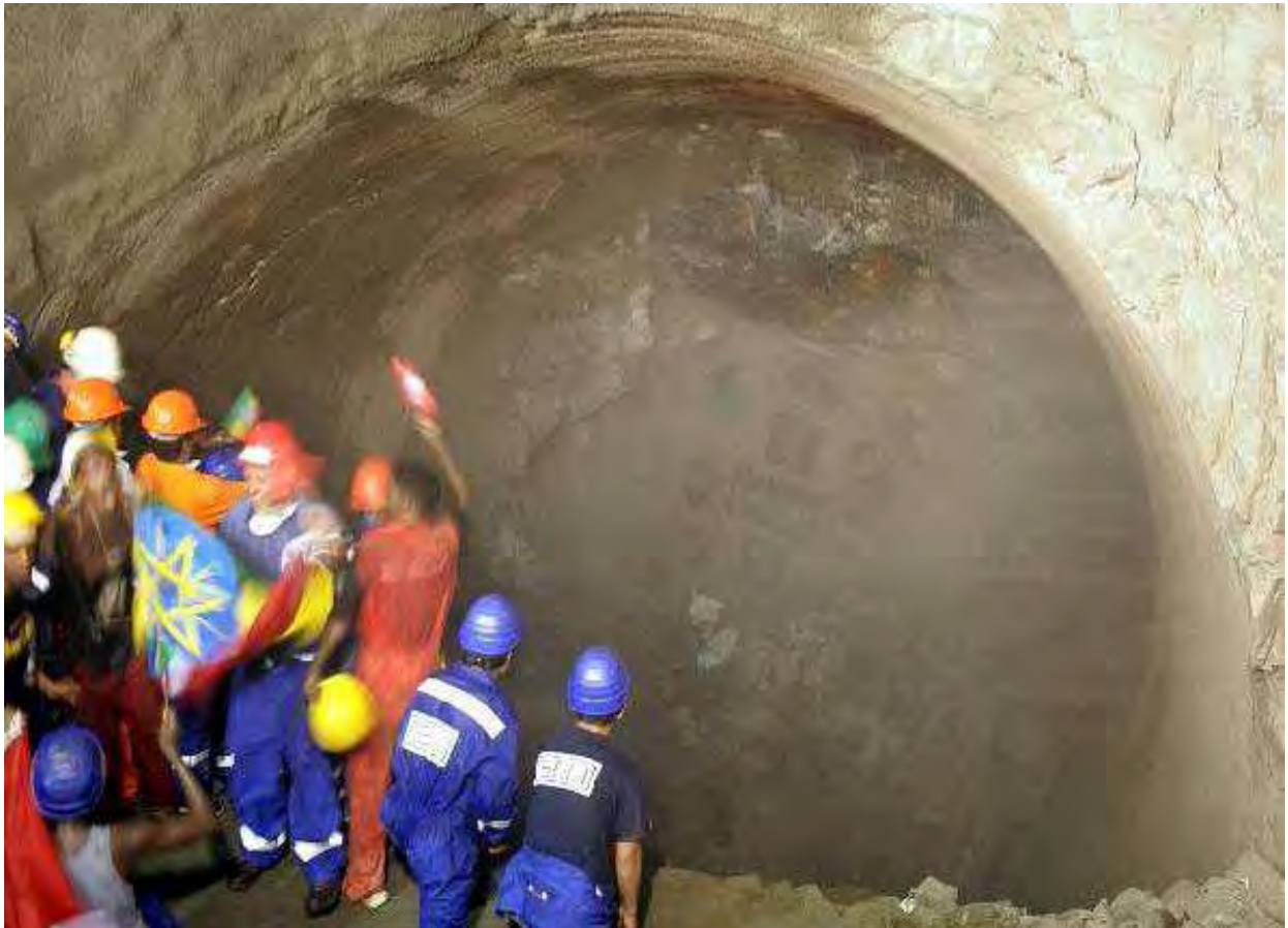
Figure II - 17: Breaking the final tunnel diaphragm 06.2009 Source: doc. photo Salini
