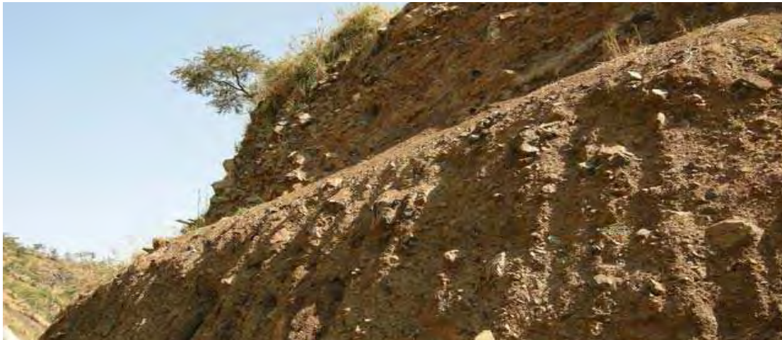
Figure III - 37: Road cutting covered by alteration with a sandy loam grain with brecciated materials Source: doc. EEPCo - ELC Report, 12.2007
