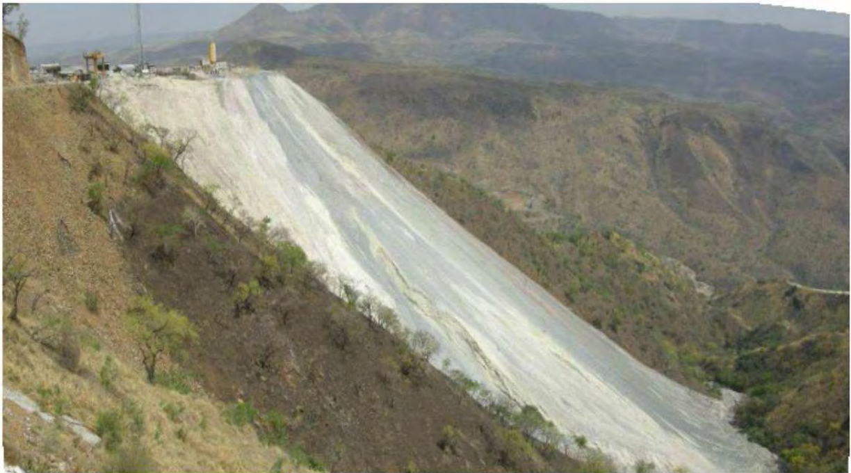
Figure III - 40: Tunnel excavation debris disposal area - outlet side Source: ELC, February 2009
