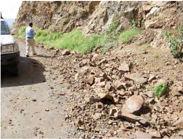
Figure III - 32 Fall of breccia onto the road Source, Evaluation Group photographic doc., 05.2012
