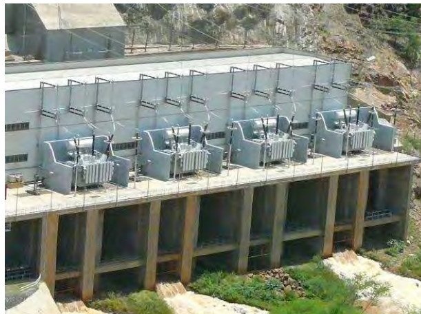
Figure II - 30: 15/400 kV transformers
