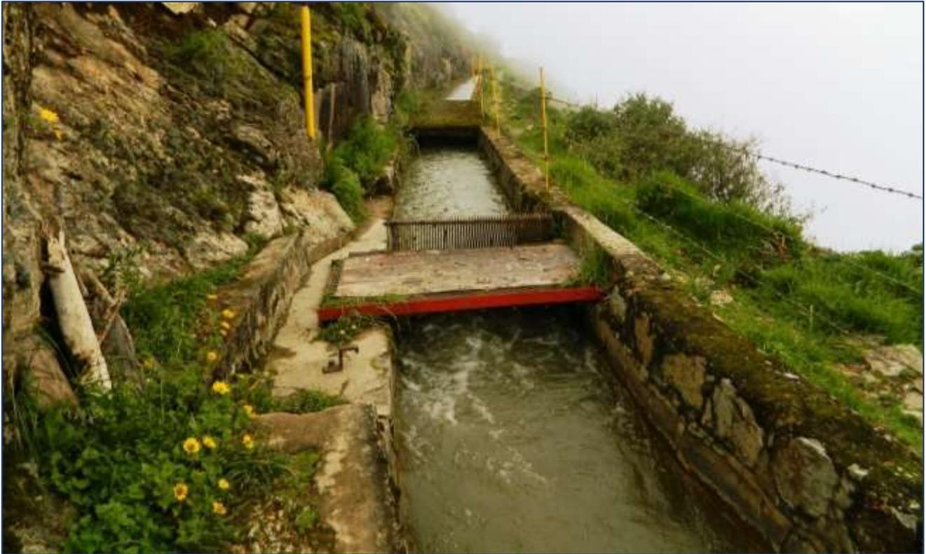
**FIGURA 3. 9: COMPONENTE PRINCIPAL: CANAL DE CONDUCCIÓN – TRAMO CERRADO**
