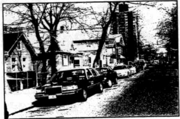
7 Rezoning Sub-Area 1: R6 to R5 West side of Corlear Avenue, north of West 230th Street.
