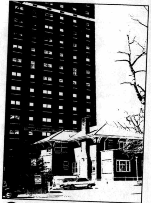
2 Rezoning Sub-Area 11: R7-1 to R-7A Completed new high-rise development at Netherland Avenue and Henry Hudson Parkway East.
