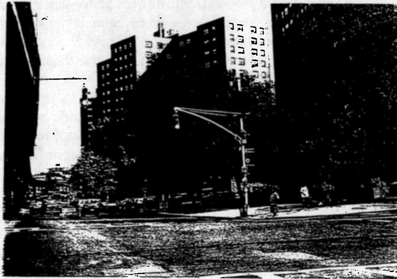
The New York City Housing Authority's Marble Hill Houses complex.
