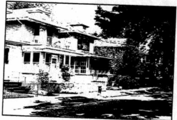
5 Rezoning Sub-Area 2: R6 to R6A West side of Sedgwick Avenue, north of Giles Place.
