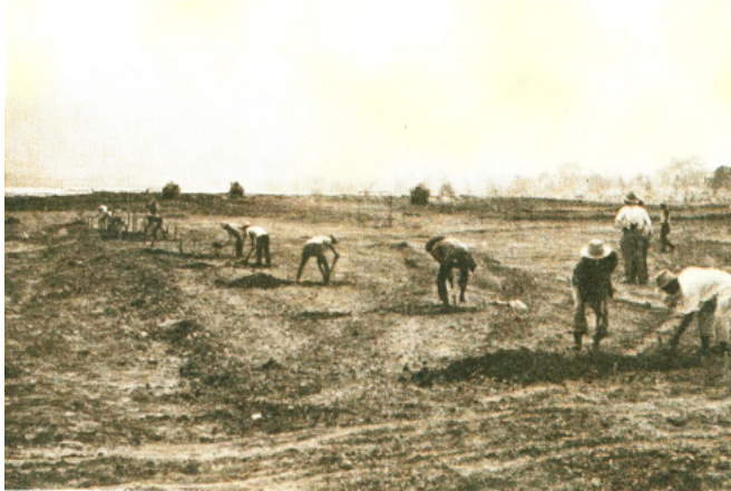
The start of construction work on IRRI's physical plant, 26 September 1960, as workers dig holes for the footings for the Service Building. In the background Higamot Hill has essentially disappeared.
