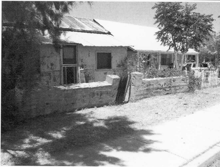
Photo 5. Unique, hand-poured wall marking the front property line of 371 E. Fifth Street. Note also the green painted house walls. Both the garden wall and the pastel color of the house walls are Mexican cultural traits.
