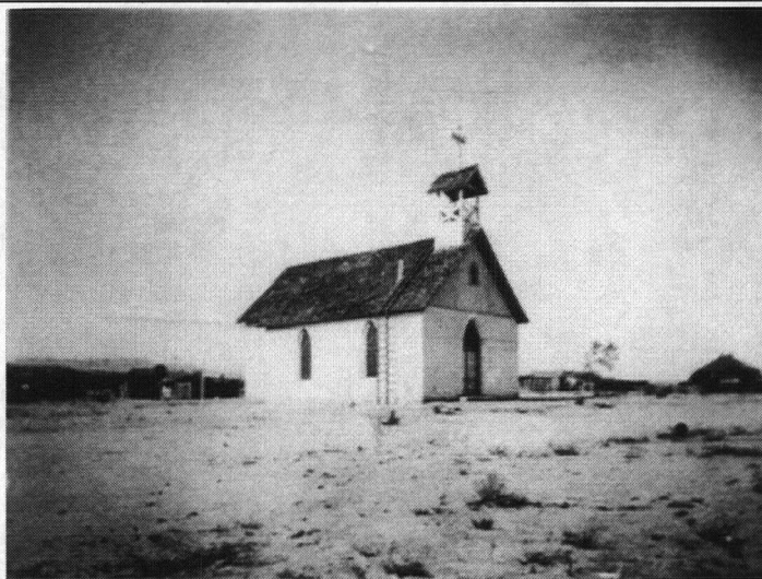
Photo 22. Our Lady of Lourdes Catholic Church, first building. Built on Block 25 in 1895, this modest, Gothic Revival-influenced adobe church served Benson and surrounds and as the heart of the Barrio, probably around 1895.
