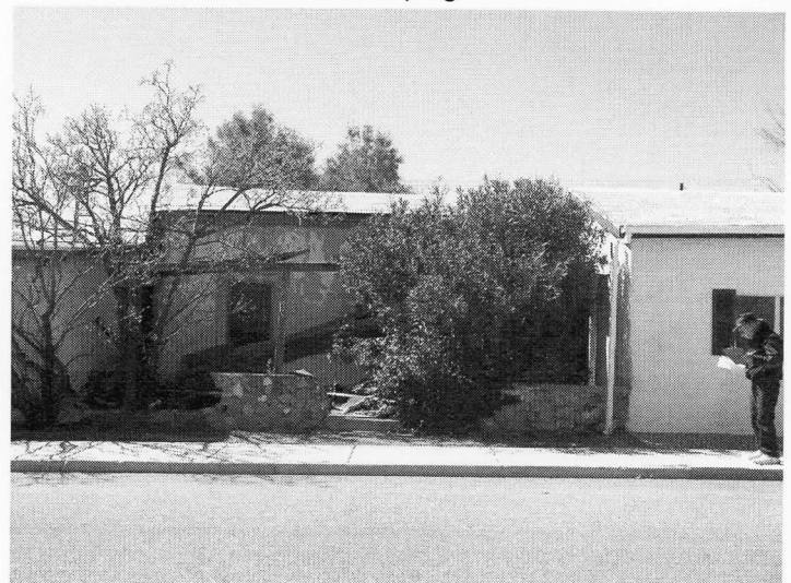
Photo 4. 478 E. Fifth Street. This transitional, side-gabled massed-plan dwelling is placed so that its walls abut those of its neighbor, a Mexican settlement trait. 464 E. Fifth Street, next door, is placed very close to the front property line.
