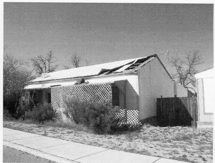
Photo 12. 463 E. 5 th Street. The 1900 Genaro Figueroa house was originally a Sonoran, parapet-walled, flat-roofed dwelling. It was later transformed by the addition of a pitched roof, exemplifying the "transitional" tradition.
