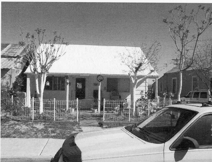
Photo 11. 387 E. Fifth Street. A second generation "railroad house" built in 1925. This is a side-gabled linear-plan type with shed additions to the rear.
