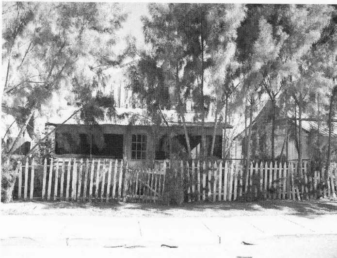
Photo 7. 369 E. Fifth Street. A 1900 "railroad house" west of Gila Street. This is a gable-front, massed-plan dwelling, a Euroamerican vernacular type. Built of frame, it may be an example of "box construction."
