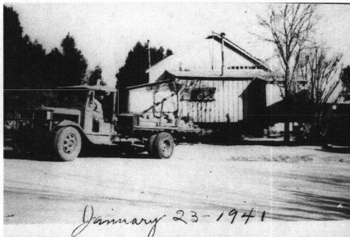
Photo 23. The home of Hi Wo's family being transported to its current location at 393 E. Fifth Street from its former location on E. Fourth Street. (The 1905 house originally came from Tres Alamos.) January 1941.
