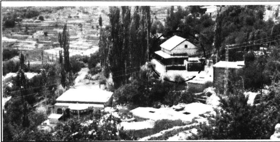
Fig. 5.3 The project site with the old jamat khana building. Photo taken in June 1986.
