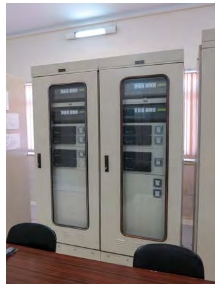
Figure 5.2-23 Transformer Protective Relay Panel
