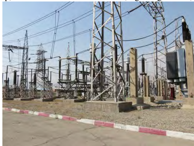
Figure 5.2-21 230kV Feeder Bay
