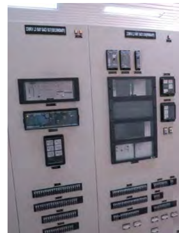
Figure 5.2-15 230kV Transmission Line Protective Relay Panel
