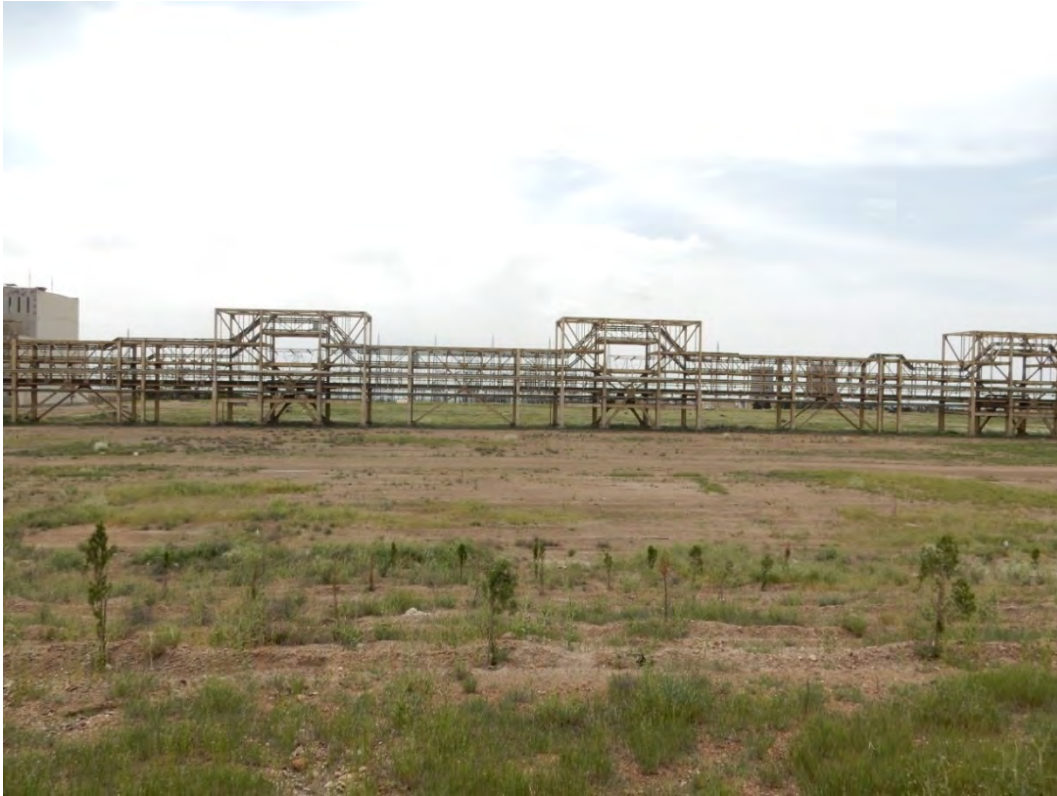
Figure 5.3-3 CASE-1 West Side Installation Space Photograph
