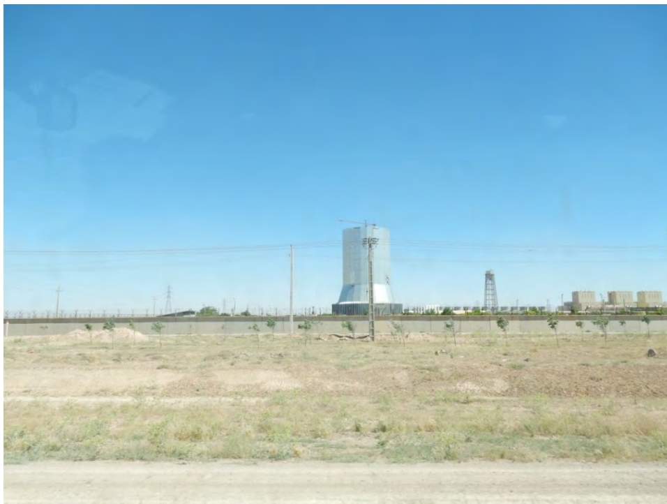
Figure 5.1-7 Shahid Mofatteh Power Plant (Dry Cooling Tower & 250 MW × 4 Units)
