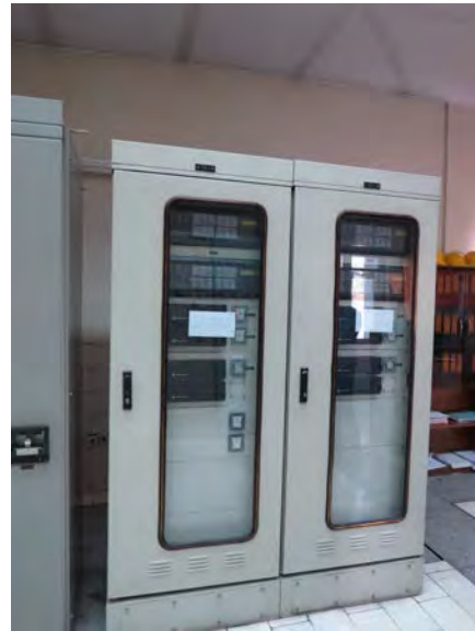
Figure 5.2-26 Transformer Protective Relay Panel
