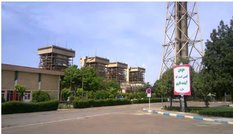
Figure 5.1-3 Shahid Rajaei Power Plant 1,000 MW (250 MW \times 4 Units)
