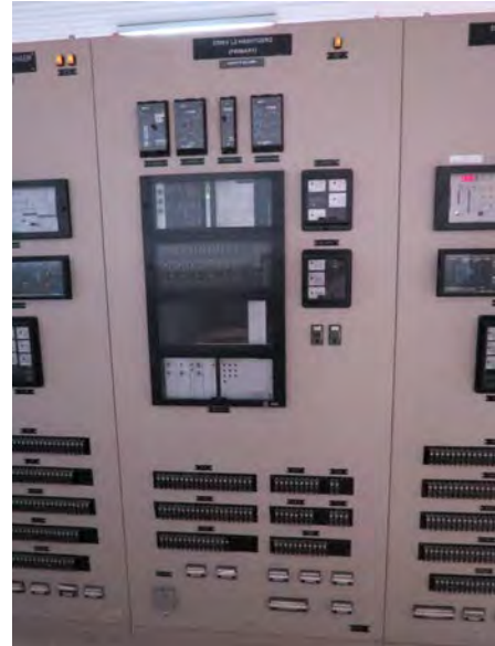
Figure 5.2-20 230kV Transmission Line Protective Relay Panel
