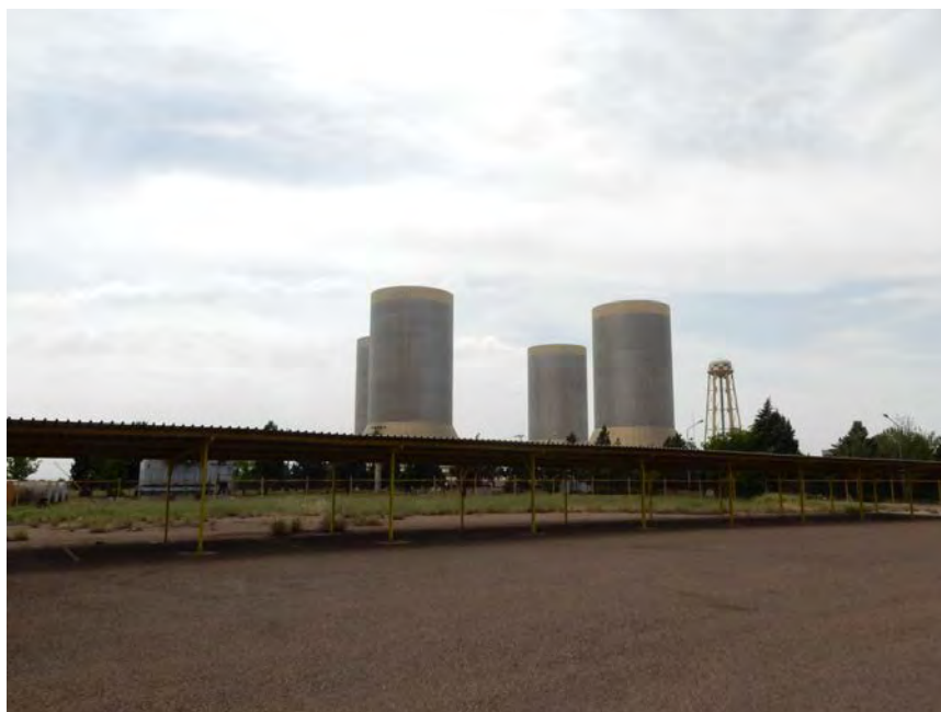
Figure 5.1-4 Shahid Rajaei Power Plant (Dry Cooling Tower)
