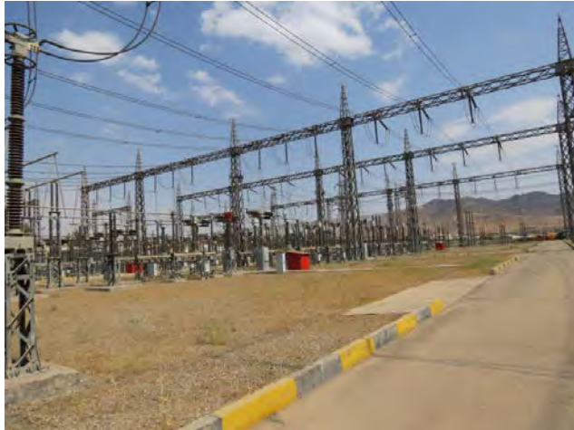
Figure 5.2-4 230kV Switchgear
