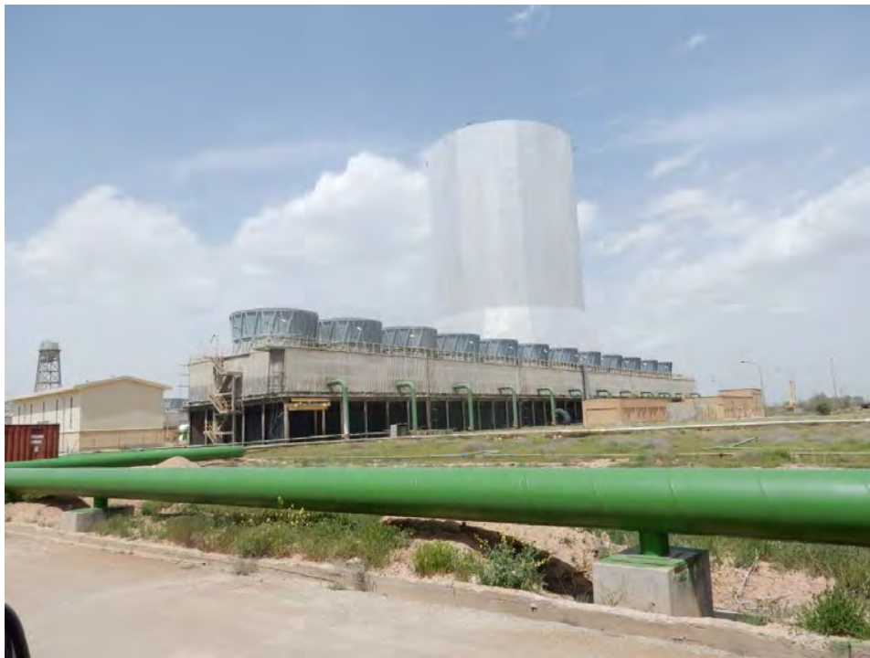
Figure 5.1-8 Shahid Mofatteh Power Plant (Wet Cooling Tower & Dry Cooling Tower)
