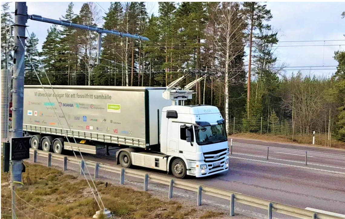
Figure 20: An eHighways truck with current collector on pentagraph and overhead lines.
