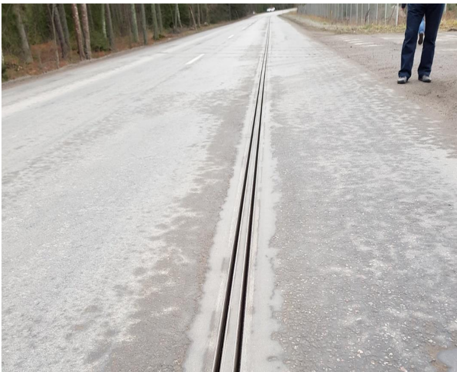
Figure 22: Rail in the road at Rosersberg, with narrow spacing, Sweden.
