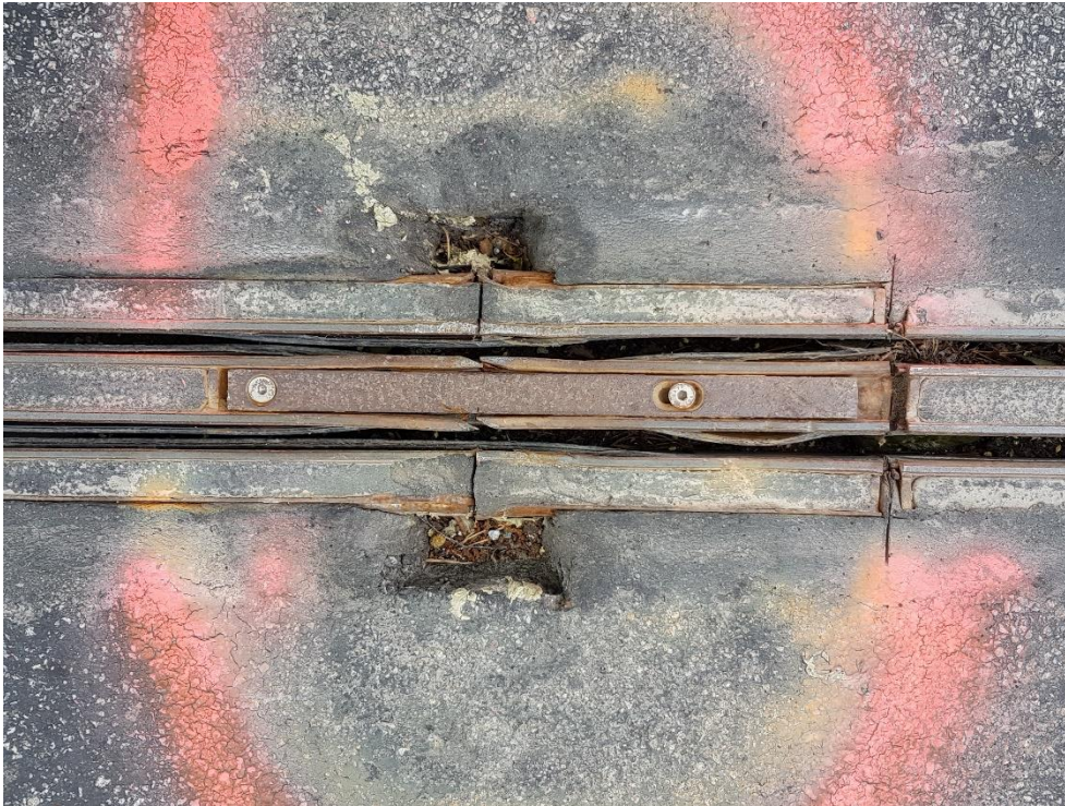
Figure 23: Joint between ERS units (Photo by Terence McGarvey).
