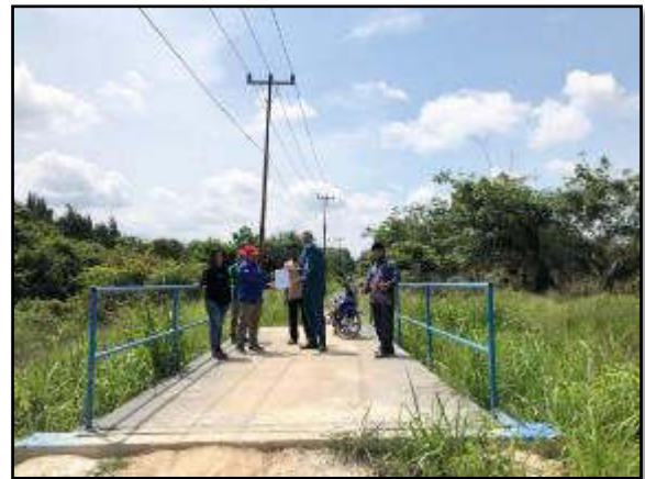
Figure 5.4-8: Bridge at Tenayan post-construction
