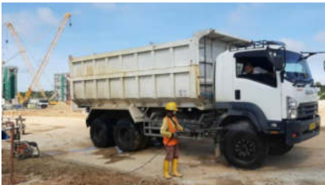
Figure 8.6-3: Wheel Cleaning at Wheel Washing Facilities at Power Plant Site
