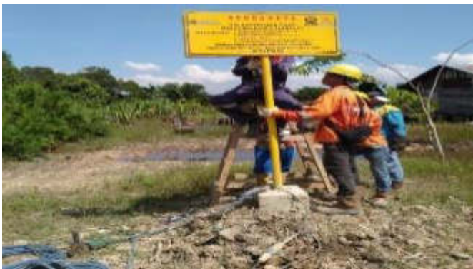
Figure 8.16-4: Warning Sign Board Installation at Gas Pipeline Route KP 01+500
