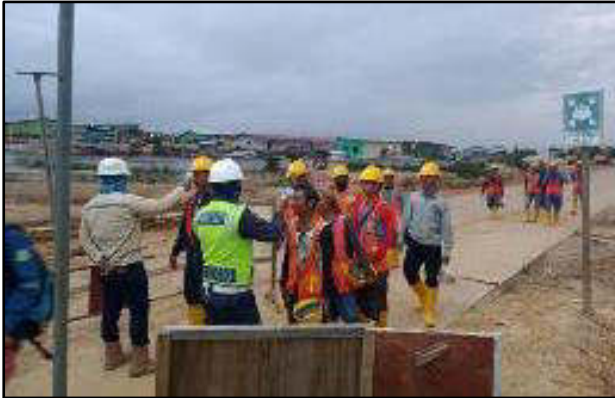
Figure 8.15-1: Workers temperature check
