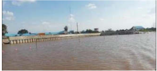
Figure 8.6-2: Silt curtain in place during dredging activity at temporary jetty
