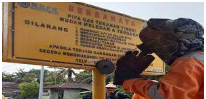
Figure 3.2-3. Installation of Warning Sign Board along Gas Pipeline Route
