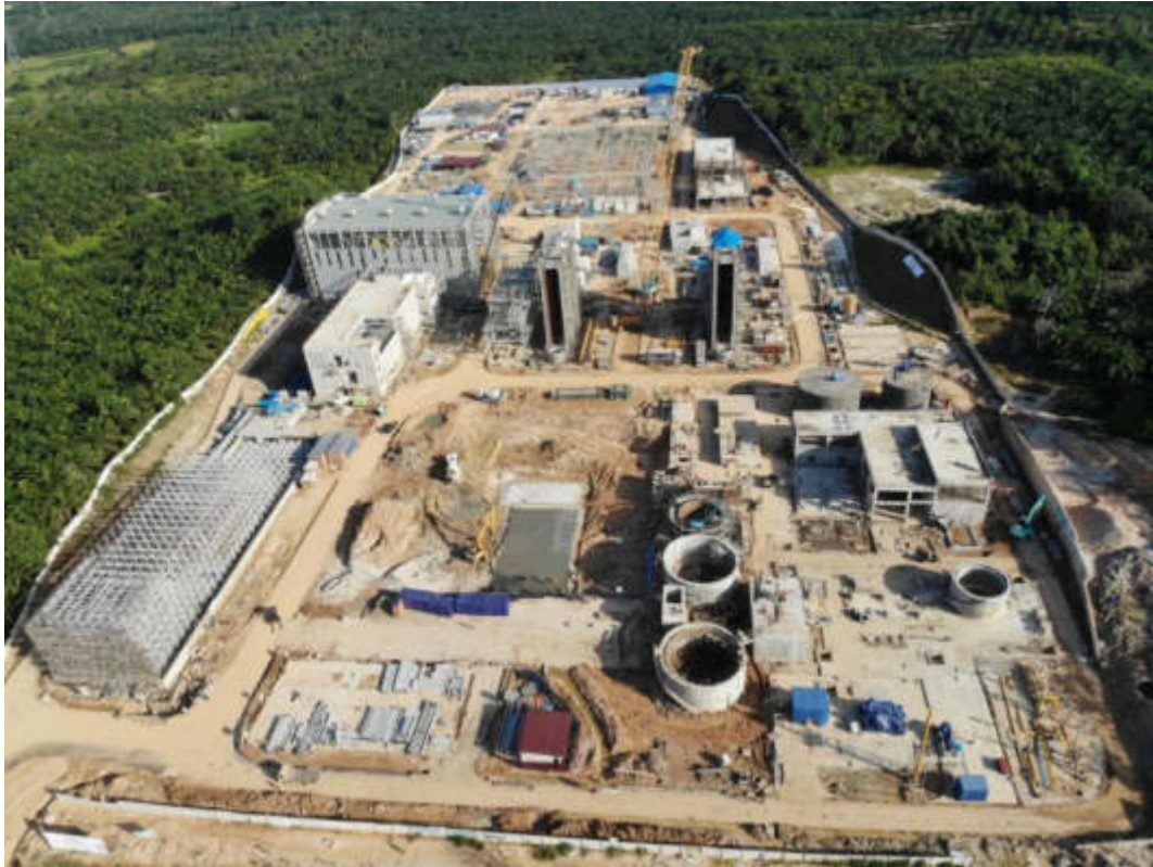
Figure 8.13-1. Fencing Around the Power Plant Site
