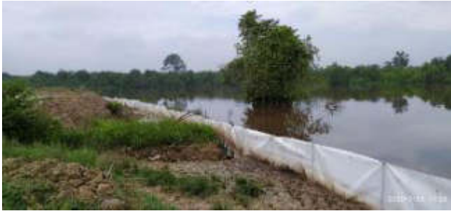
Figure 8.6-1: Silt fencing at the temporary jetty area
