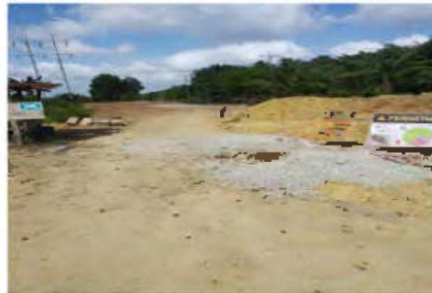
Excavation pit beside access road for people nearby
