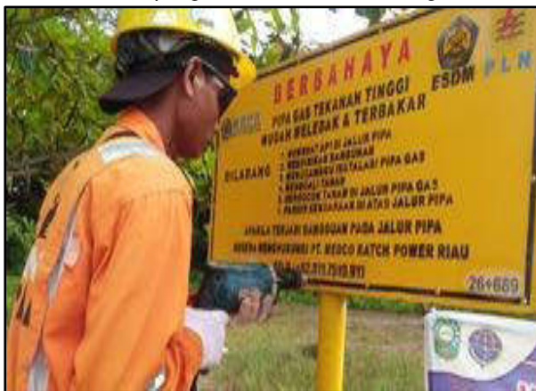
Figure 5.5-1: Sign board is being installed
