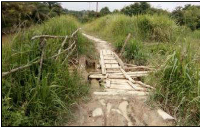
Figure 5.4-7: Bridge at Tenayan pre-construction
