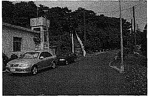
▲要往風力塔及觀測坪的階梯
