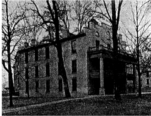
East Wing, First Home of Civil Engineering
