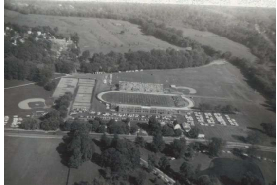
Peden Stadium prior to Hocking Relocation
