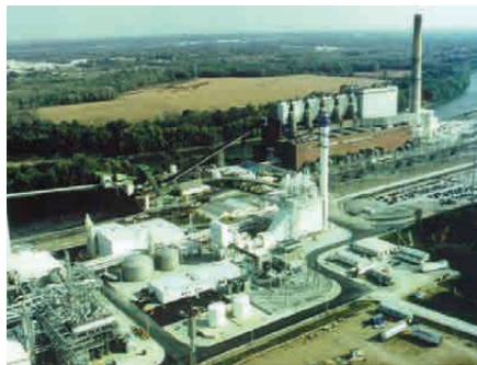
View of the Wabash River Generating Station. The new section of the plant, comprising the coal gasifier, gas-purification system, and a gas turbine, is in the foreground; the old section, containing the steam-powered component of the IGCC process, stands at the upper right.
