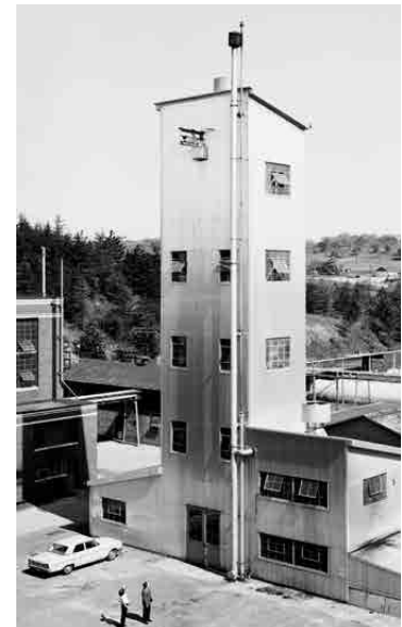
Pilot plant at Bruceton for testing the alkalized-alumina process of removing sulfur dioxide from the flue gas of coal-burning boilers. (photo credit: National Archives and Records Administration)
