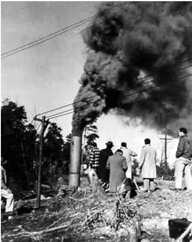
Minutes after the initial fire was lit at Gorgas, billowing smoke revealed the progress of underground coal combustion and gasification. (photo credit: National Archives and Records Administration)
