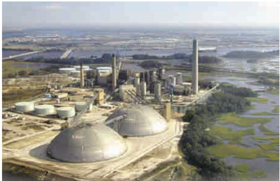
JEA clean coal plant in Jacksonville, Florida.
