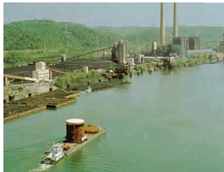
A barge carrying the pressure vessel for the country's first commercial-scale demonstration of a pressurized fluidized-bed combustion boiler approaches the Tidd Station at Brilliant, Ohio, in 1989.
