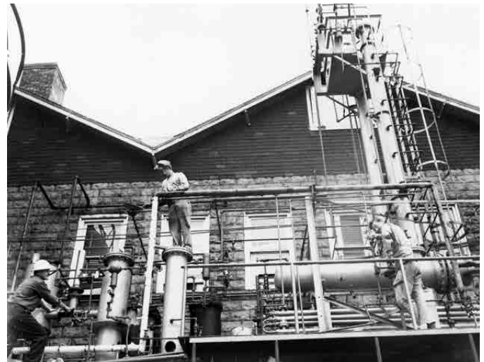
Gas-purification pilot plant under construction at Beechurst Avenue.
