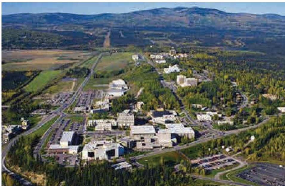
The Alaska Energy Office, a partnership between NETL and the University of Alaska-Fairbanks (UAF), is located on the UAF campus.
