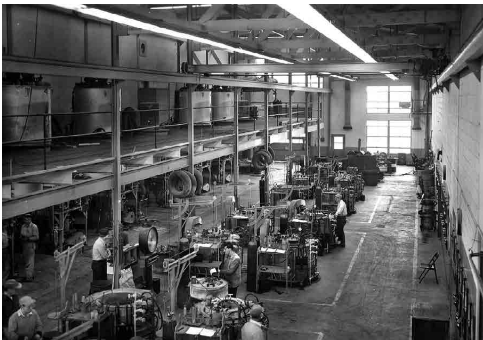
Full-scale zirconium production underway in Building 28 at Albany, 1953.
