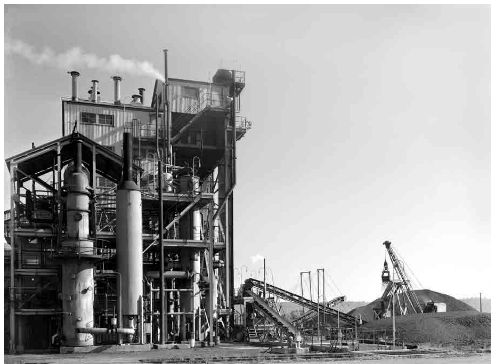
The Fischer-Tropsch demonstration plant at Louisiana. On the left side of the plant, the leftmost of the two tall cylinders is the “Morgantown-type” vertical gasifier. (photo credit: National Archives and Records Administration)
