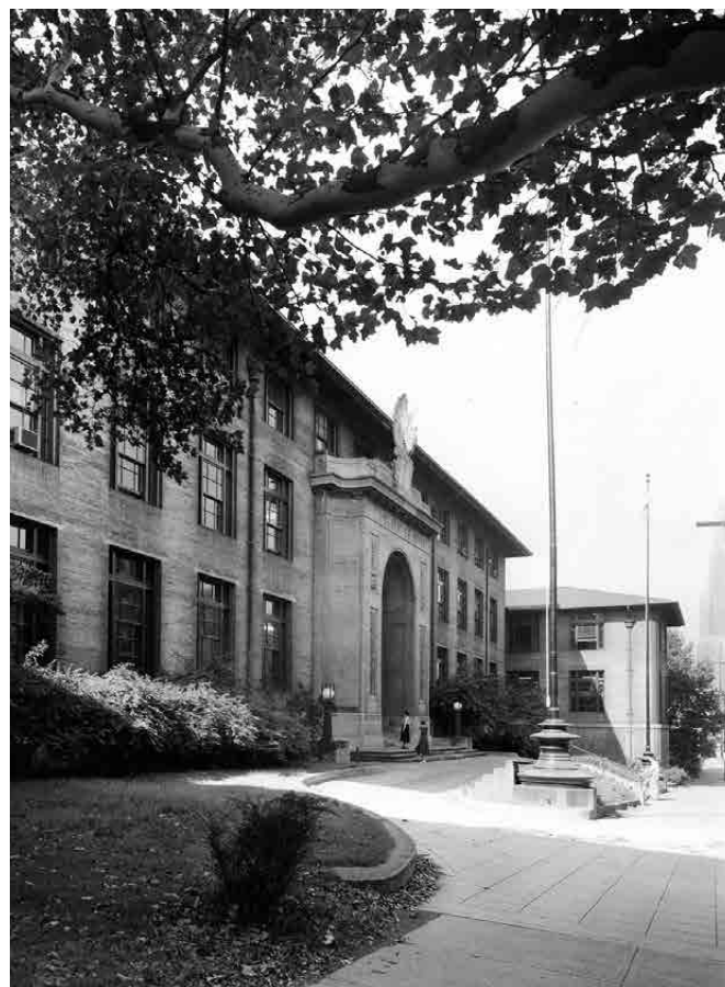
Entrance to the main building of the Pittsburgh Central Experiment Station
