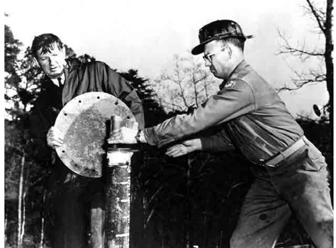
Wilburn C. Schroeder (left), chief of the Office of Synthetic Liquid Fuels, assisting as an incendiary device is dropped into a shaft to start the first underground coal gasification experiment at Gorgas, Alabama, in January 1947. (photo credit: National Archives and Records Administration)
