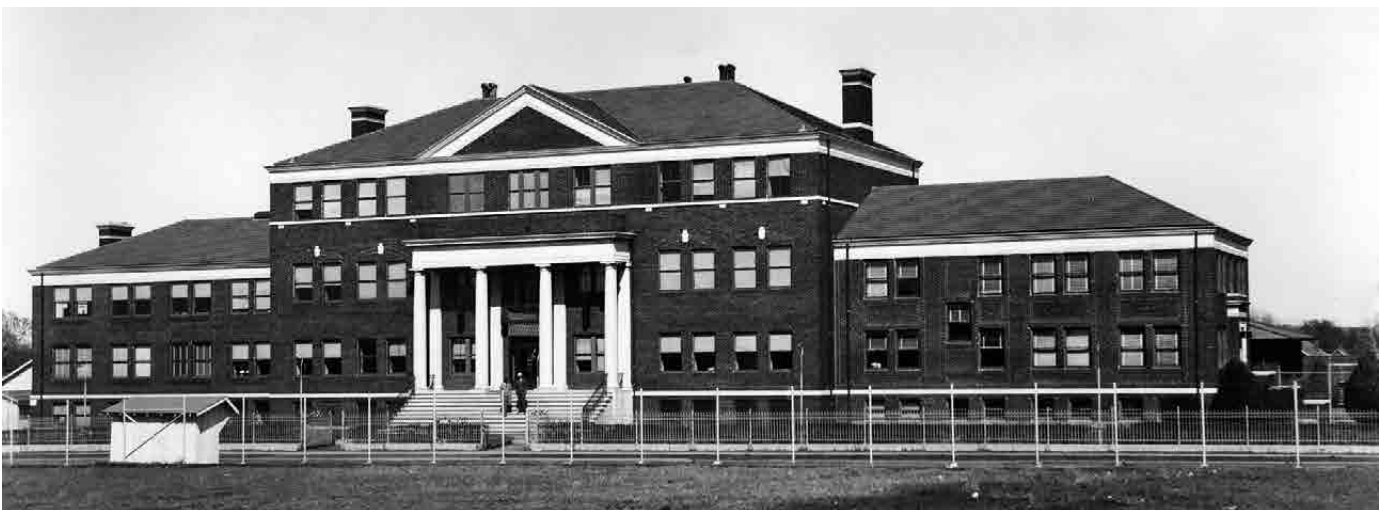
The new administration and research building at Bartlesville in 1937, built by the Public Works Administration.
