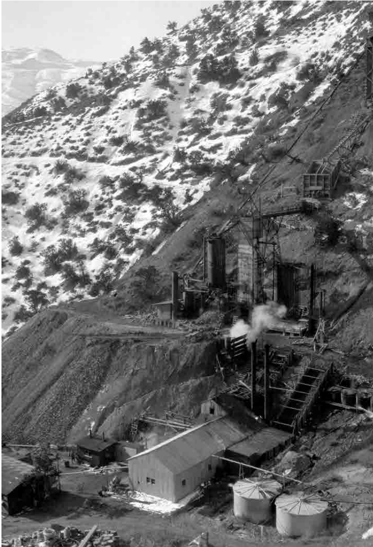
Oil-shale processing plant at Rulison, 1927. The rectangular structure at the center-right housed the Pumpherston retort, while the dark-colored cylinder immediately to its left was the N-T-U retort. (photo credit: National Archives and Records Administration)
