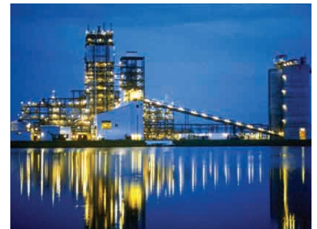
View of the Polk Power Station.
