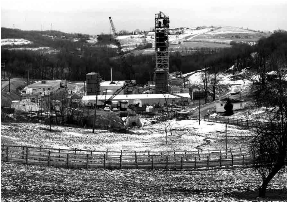
The Synthane demonstration plant under construction at Bruceton, December 1973.
