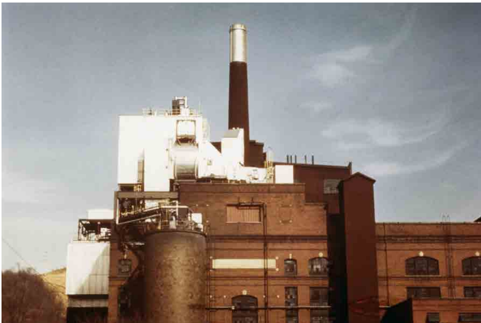
Rivesville Station, site of the first industrial-scale demonstration of fluidized-bed combustion in the United States.
