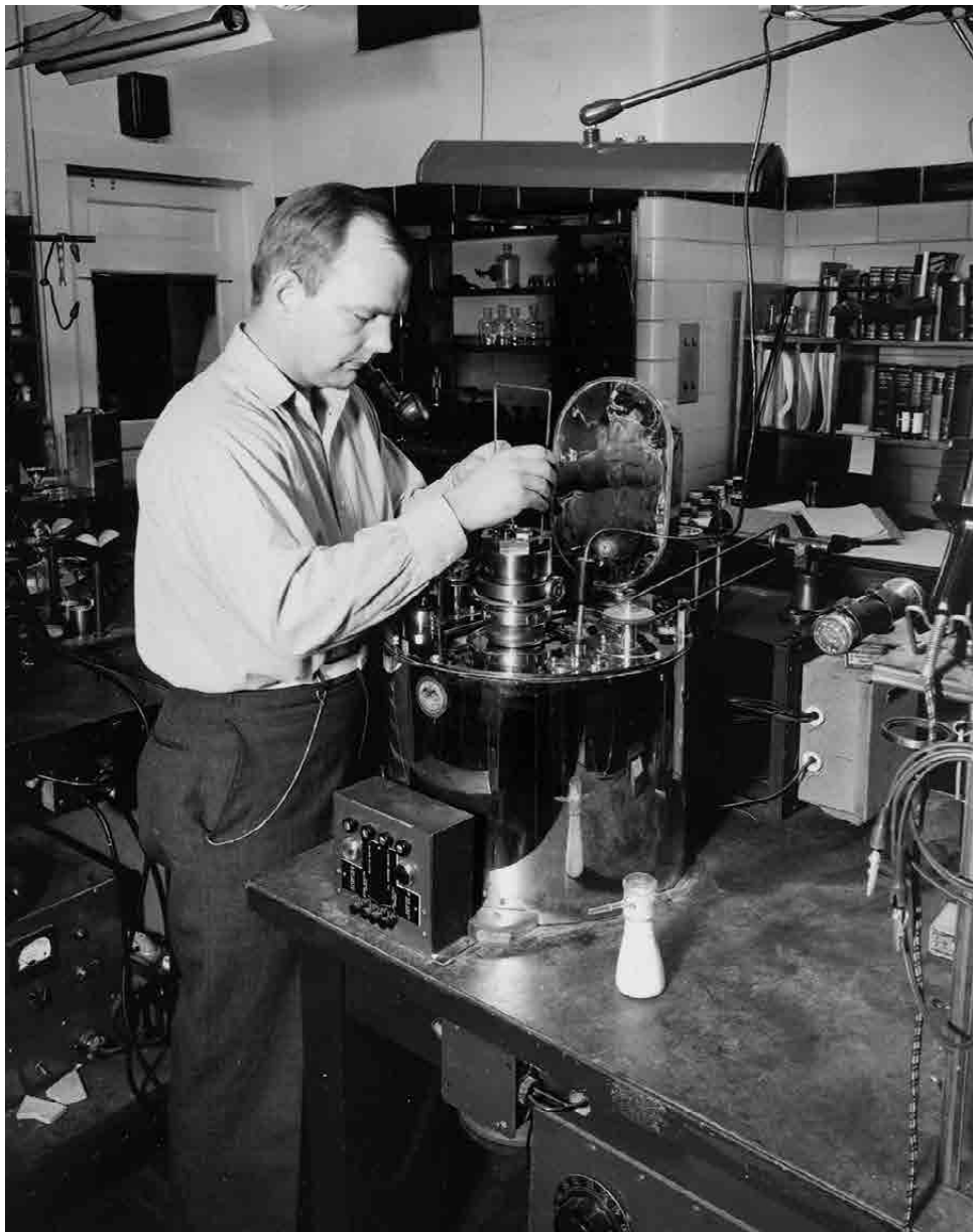
Bartlesville scientists invented the rotating bomb calorimeter to obtain precise measurements of thermodynamic properties.
