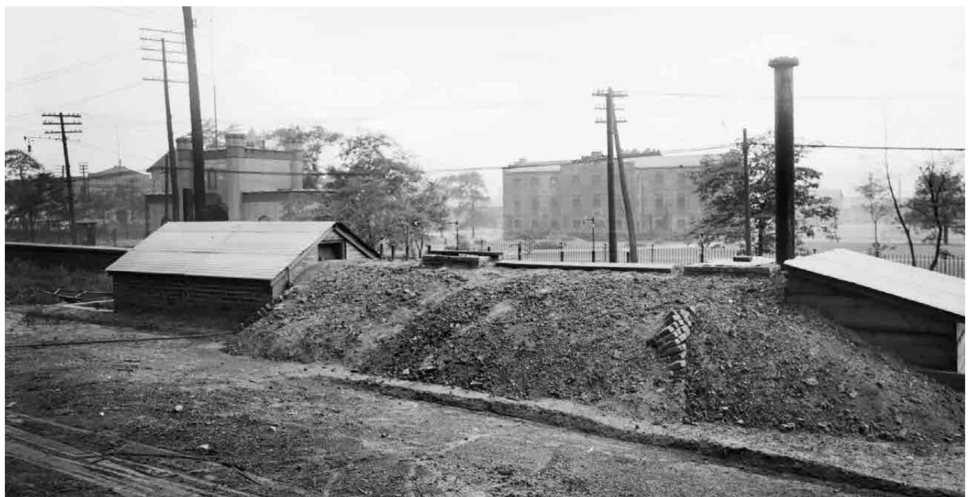
External view of mine fire gallery at the Arsenal Station.
