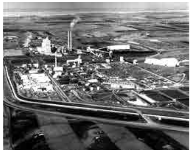
The Great Plains Coal Gasification Plant at Beulah, North Dakota. (photo credit: U.S. DOE)
