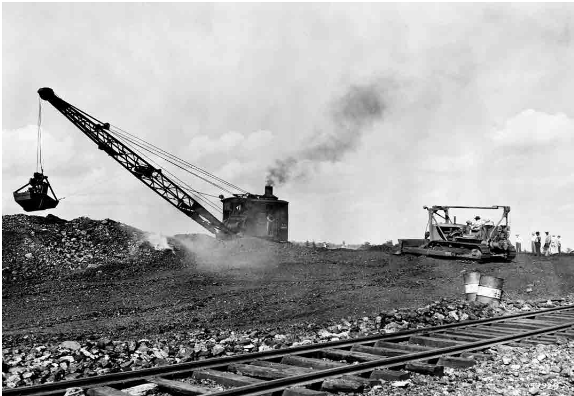
Spontaneous combustion of improperly stored coal caused this fire at the Nonconnah Yards of the Illinois Central Railroad near Memphis, Tennessee. Preventing such dangerous and wasteful fires and improving methods of extinguishing them were important missions of the Bureau of Mines during World War II. (photo credit: National Archives and Records Administration)
