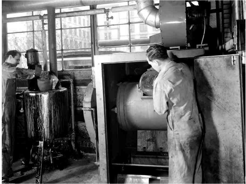
Preparing a mixture of powdered coal and heavy oil for the experimental coal hydrogenation plant at Pittsburgh. (photo credit: National Archives and Records Administration)
