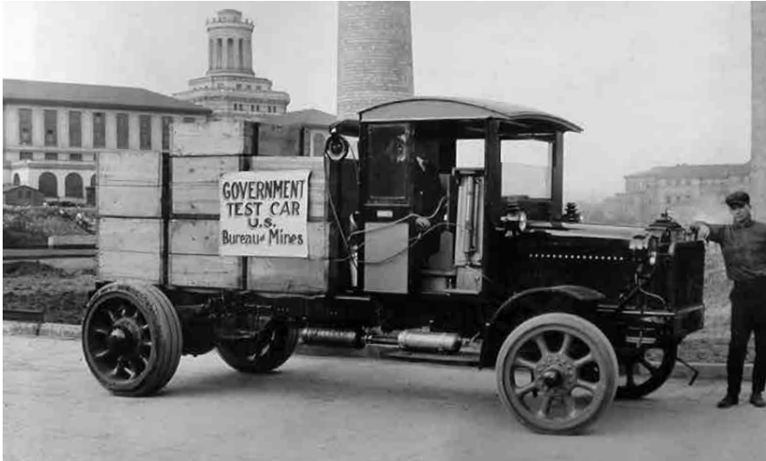
A Brockway five-ton truck participating in the Pittsburgh road tests that yielded vital data on motor-vehicle exhaust emissions. (photo credit: National Archives and Records Administration)
