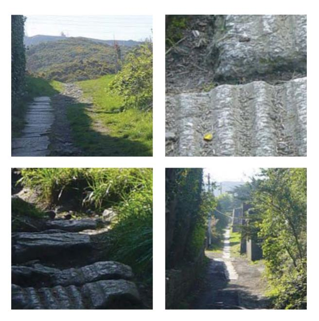
Photographs taken in 2003 of the remains of "The Flags" pathway (off Dalkey Avenue) down which the funicular railway came from Dalkey Quarry. Granite stones still in the quarry show the erosion caused by the chains which pulled the wagons.
