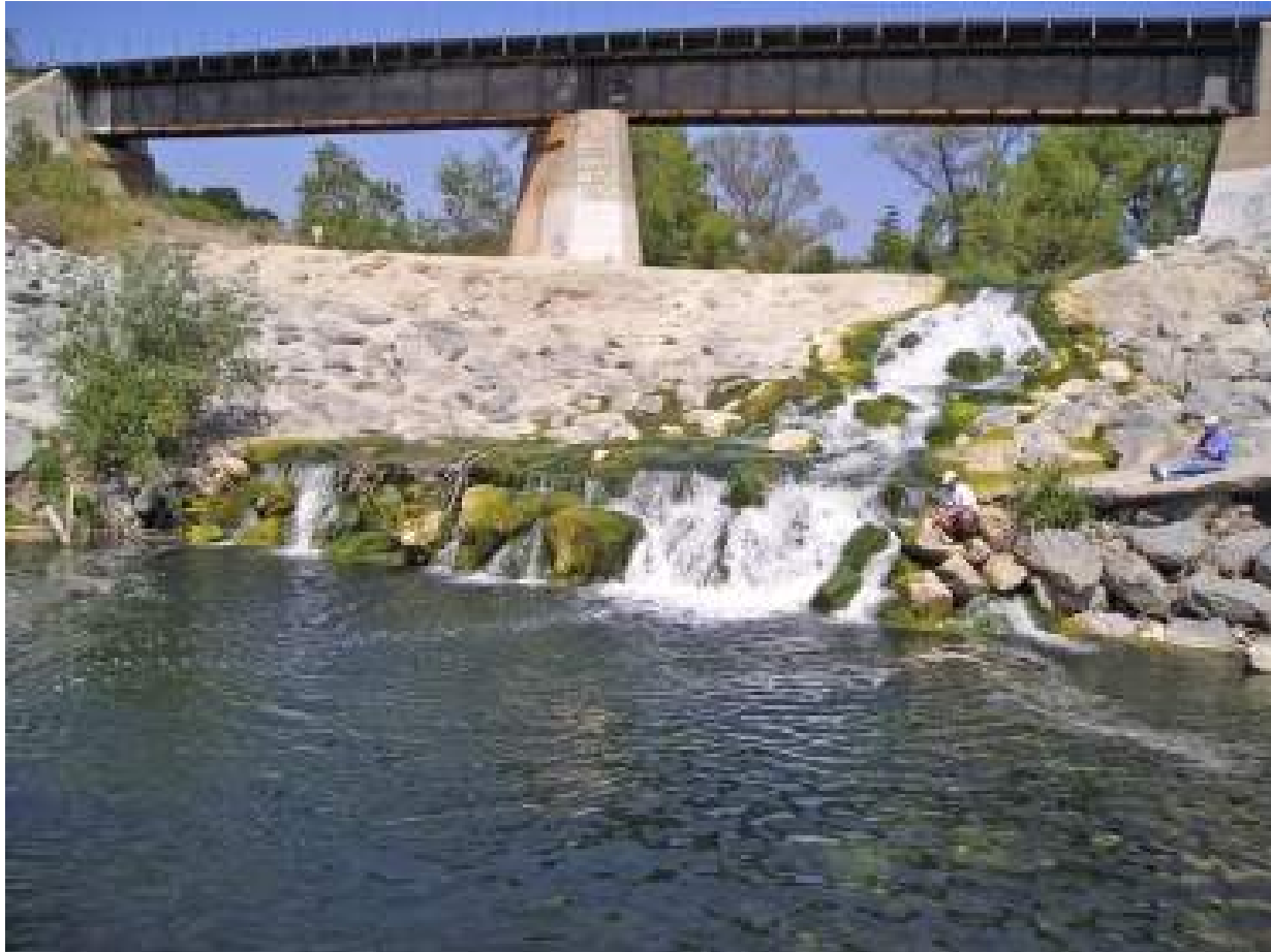
Metrolink barrier on Arroyo Trabuco Creek, tributary to San Juan Creek – 2009 Courtesy of Valerie Taylor, CDFW 4
