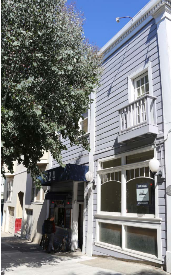
Primary façade facing Union Street, view west.
