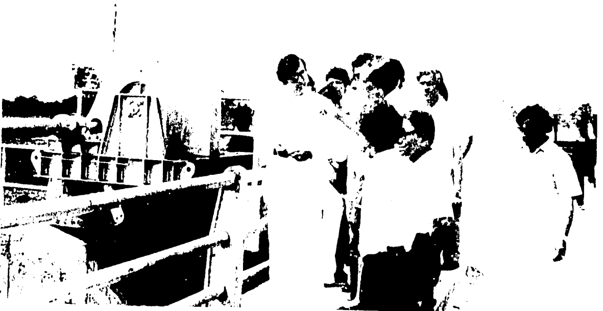
The River Valleys Development Board (RVDB) which built the Ulhitiya dam and spillway pressed into service even some Gal Oya vintage machinery, on the excavation work on the spillway to speed up work. Photograph
